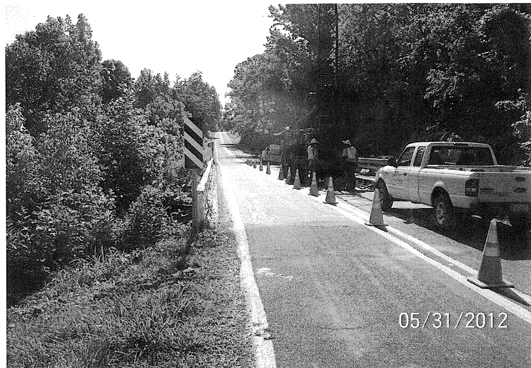
View Looking Upsation along -L- from End Bent 1
