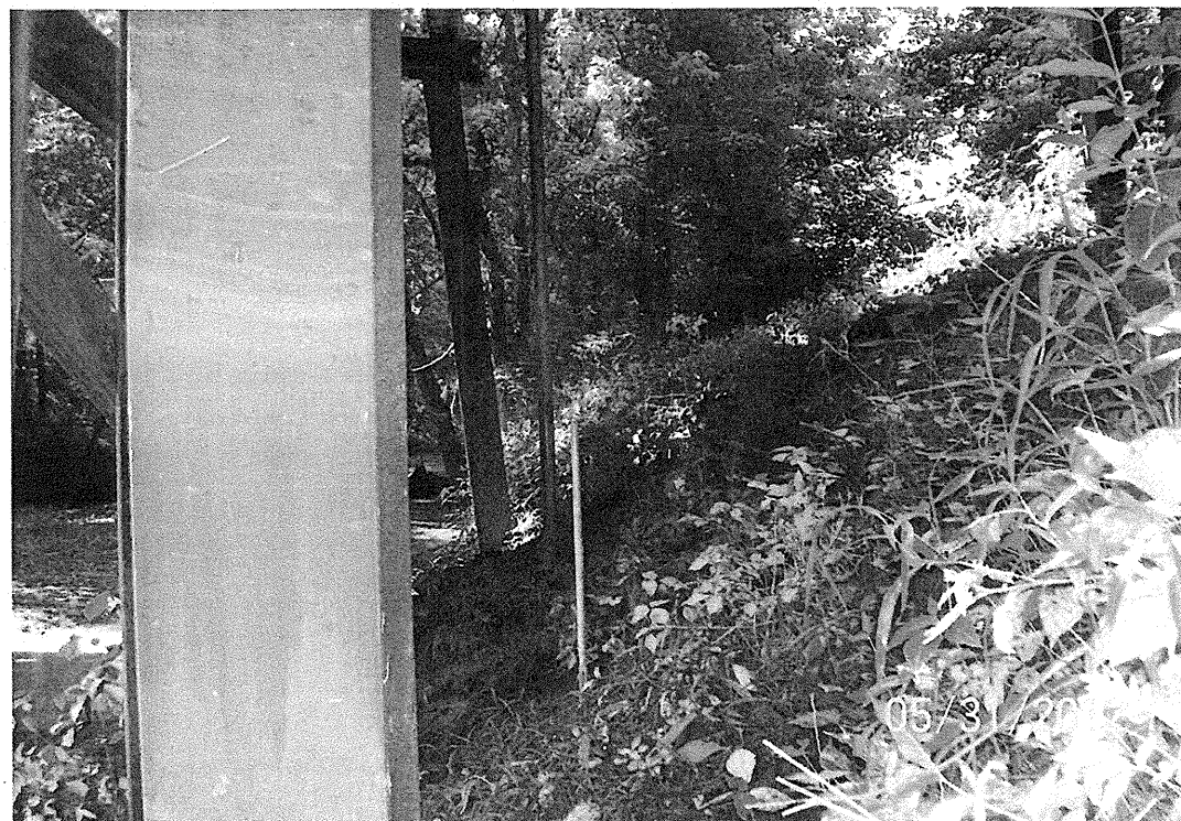
View of Bent 1 Looking Left to Right
