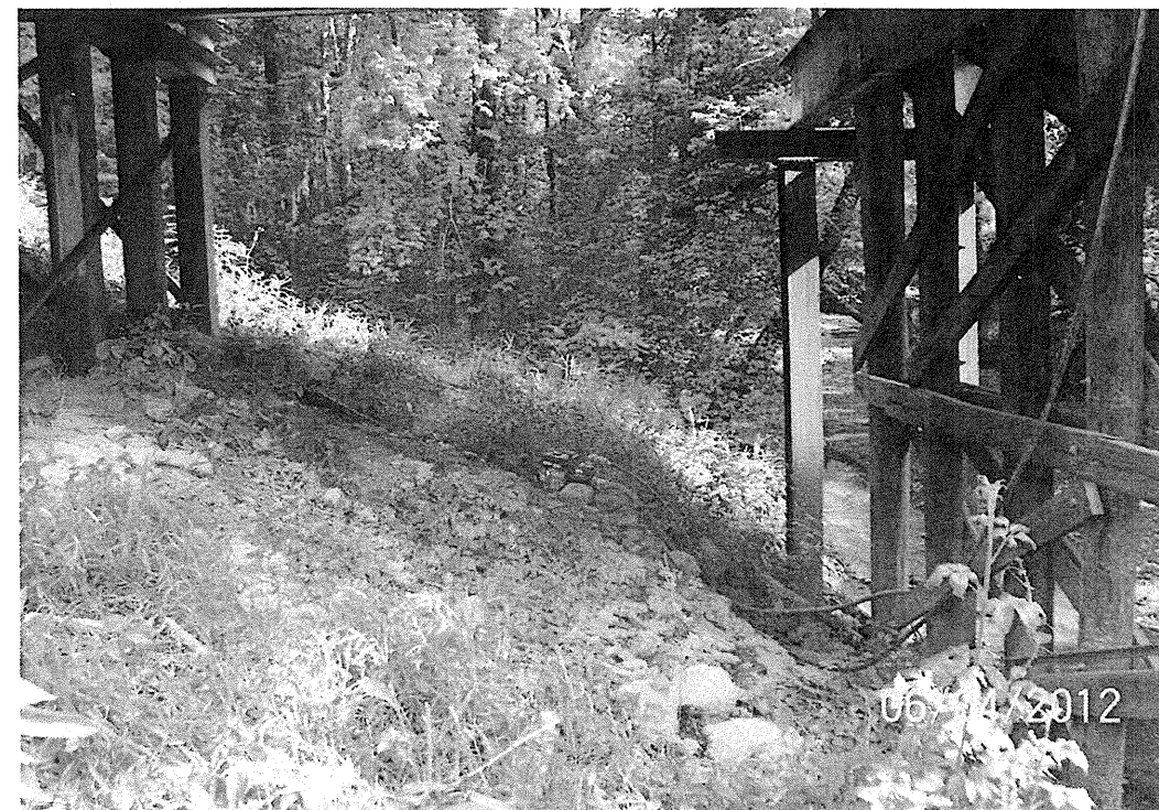
View of Bent 2 Looking Left to Right
