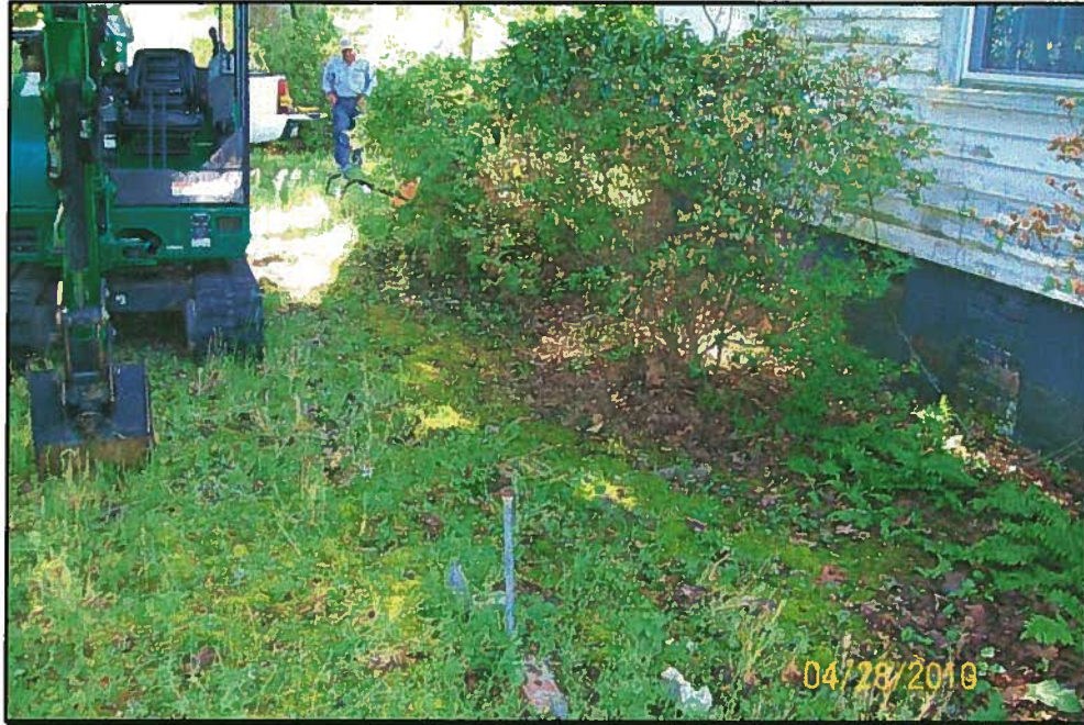
UST Location – Looking northeast along north side of former Sellers residence (note: UST piping extending above ground in foreground of picture)
