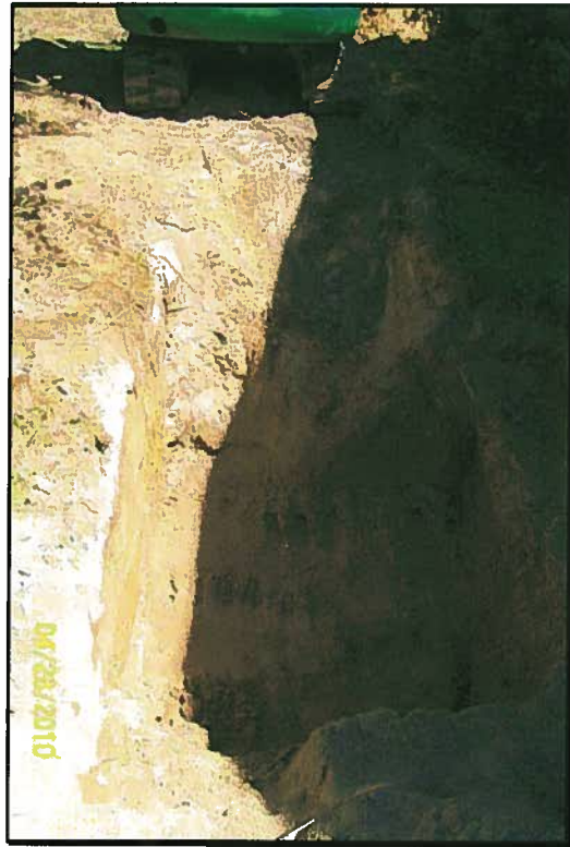
UST Excavation – Looking east across excavation from west side of excavation
