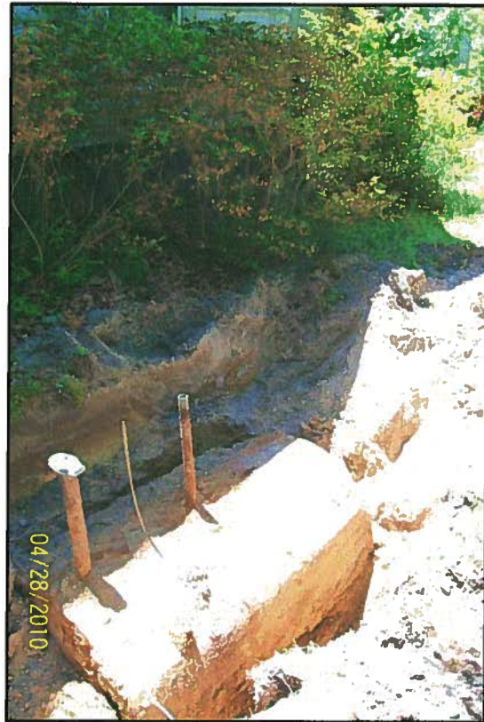
UST Excavation – Looking southwest towards northern side of Sellers residence
