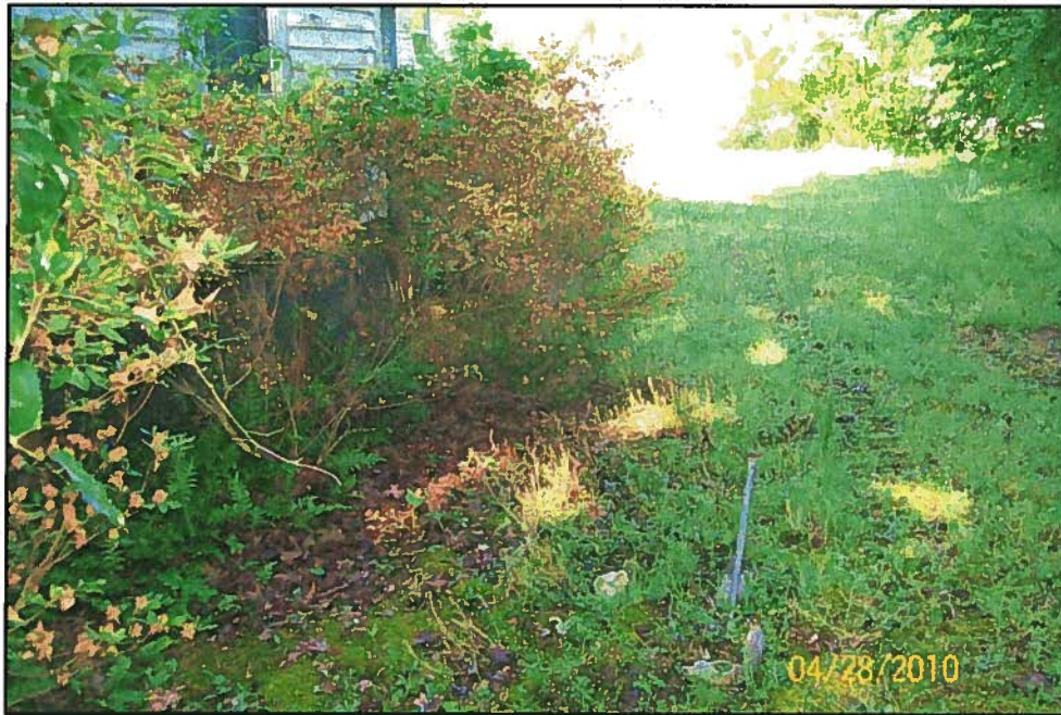
UST Location – Looking west along north side of former Sellers residence (note: UST fill port and piping extending above ground in foreground of picture)
