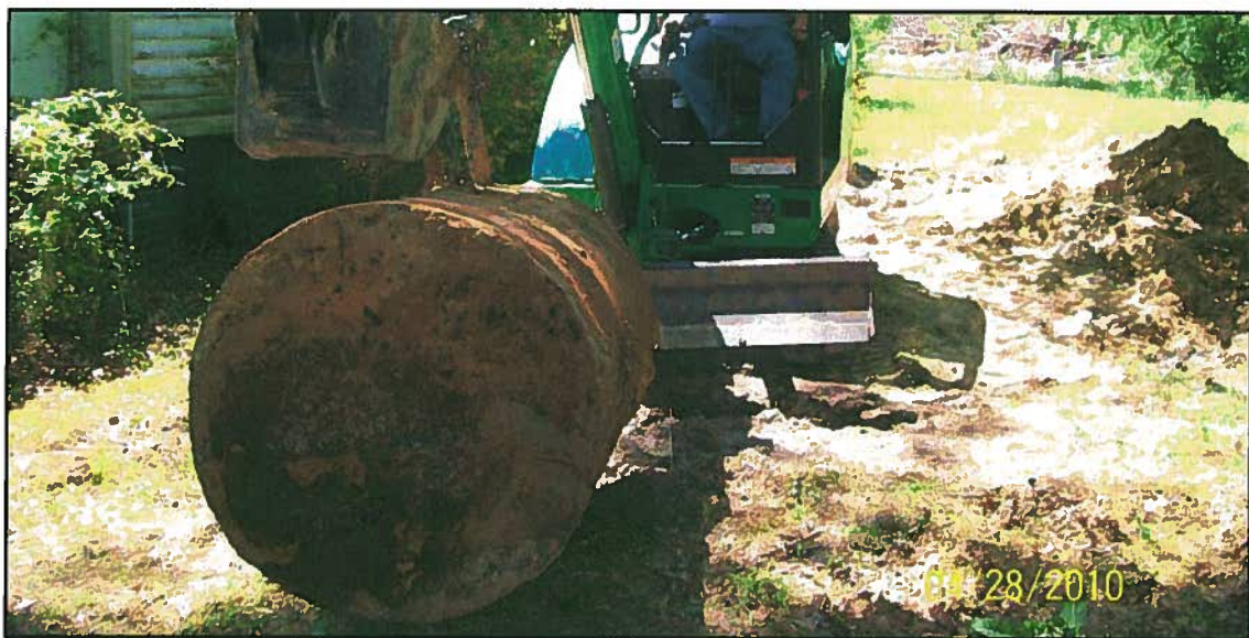
Removed UST - Looking west along north side of former Sellers residence
