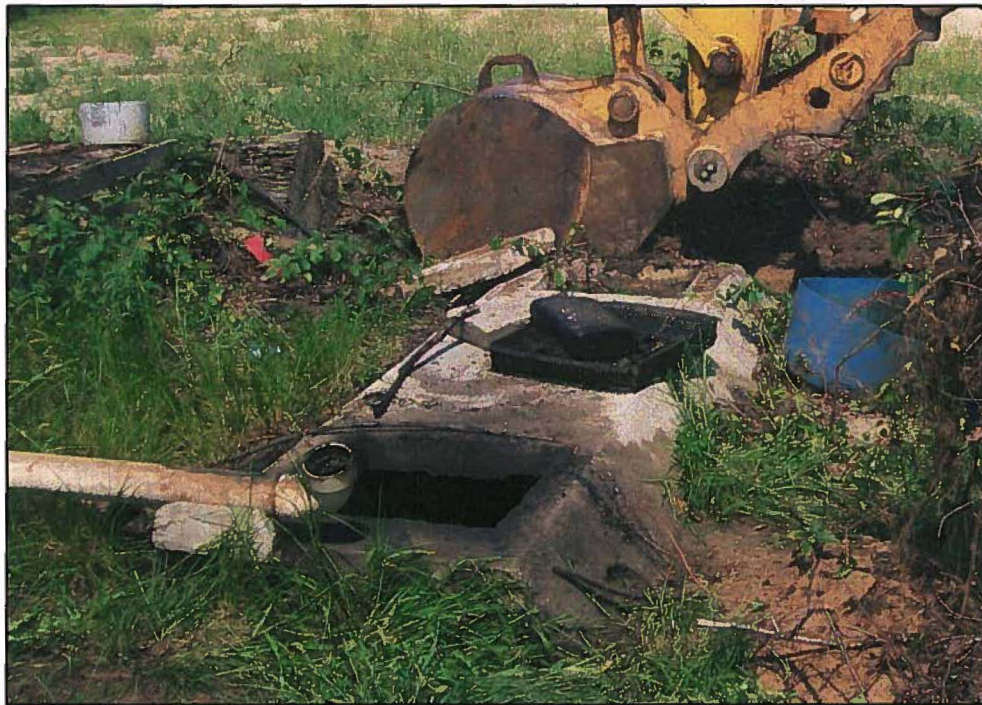
Excavating North end of oil-water separator
