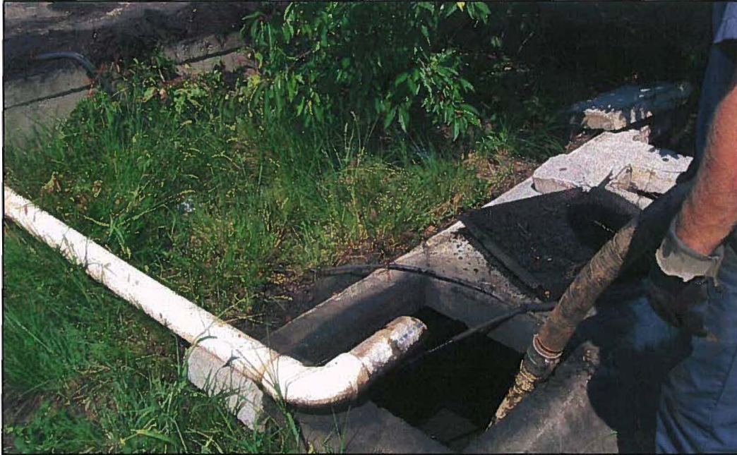
Pumping off fluids from oil-water separator
