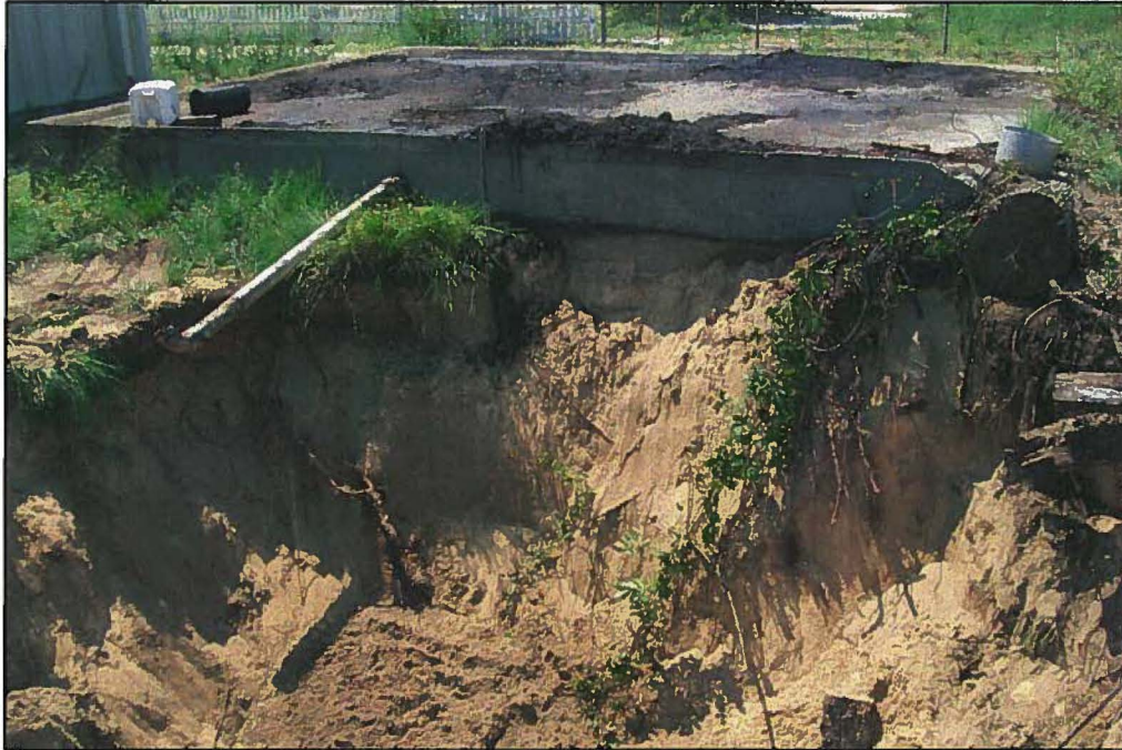
Looking Southwest across oil-water separator excavation and adjacent wash-down pad.
