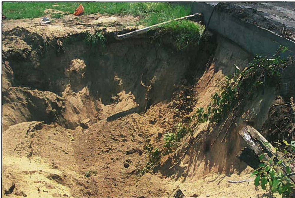
Looking South across oil-water separator excavation
