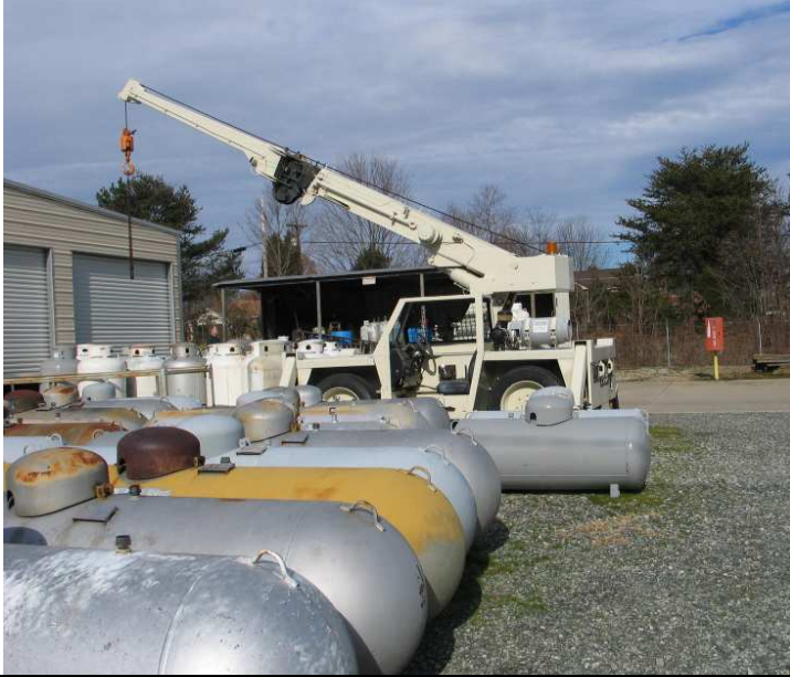
Propane tanks on east side of building.
