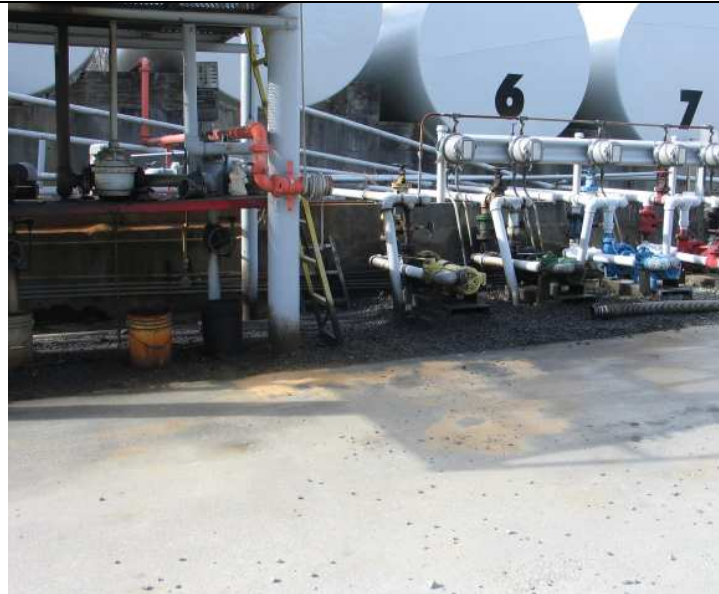
Close up of the fuel dispensing lines and valves. Note oil staining on the gravel.
