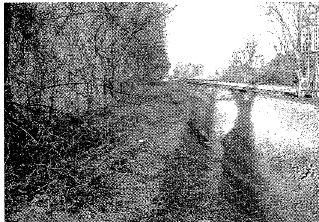
View Looking Downstation along -M1G- from End Bent 2
