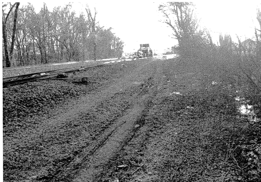
View Looking Upstation along -M1G- from End Bent 1
