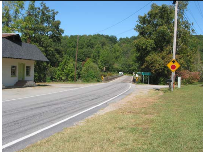
Bridge 11 on NC 175. View to the north.
