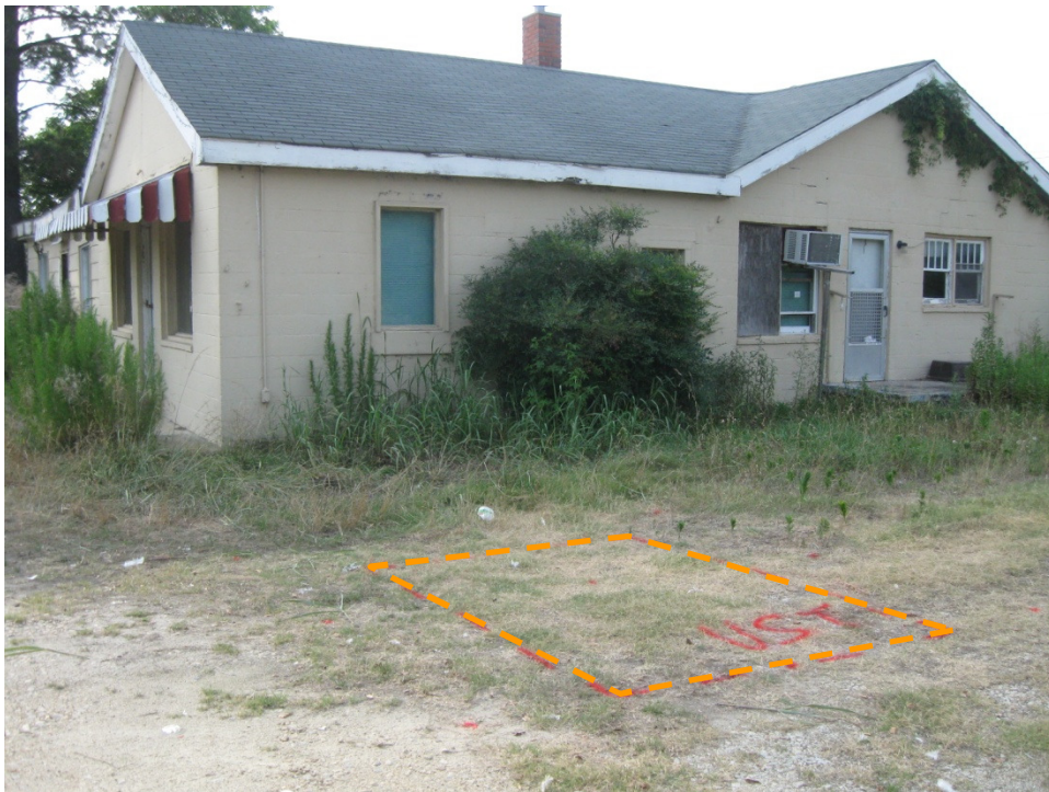
Parcel 37 – Scott McGowan Property, looking northwest. Photo shows approximate marked location of the probable UST on the east side of the property.
