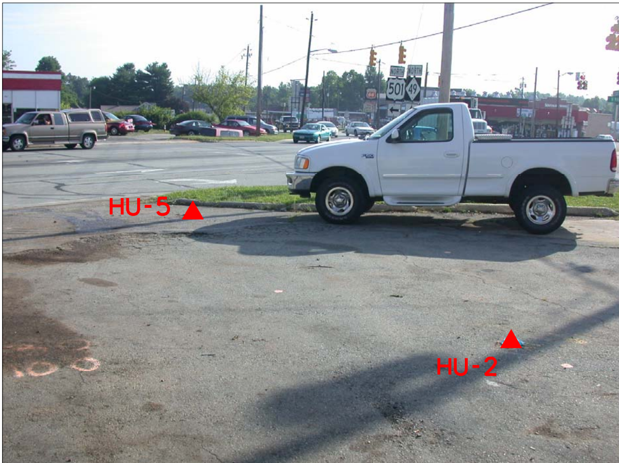
PHOTO 4 - BORINGS AT HUMPHRIES PROPERTY LOOKING NORTH FROM BUILDING
