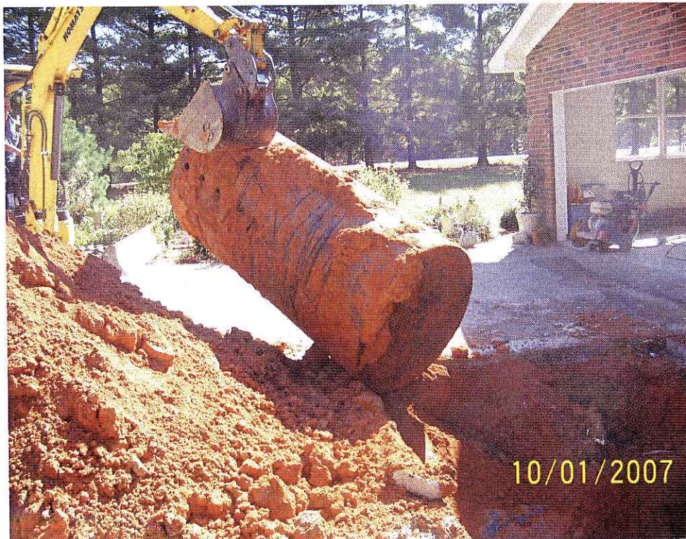
Photograph 4 - Removing the first tank from the ground.
