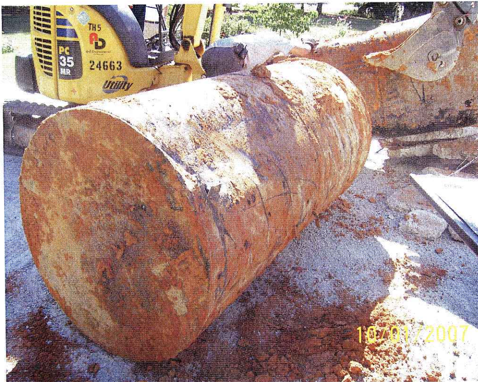
Photograph 6 – Condition of the second tank.
