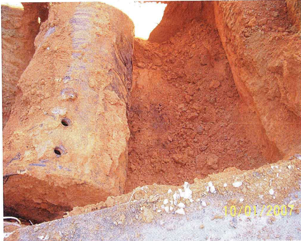
Photograph 5 – Removing the second tank.
