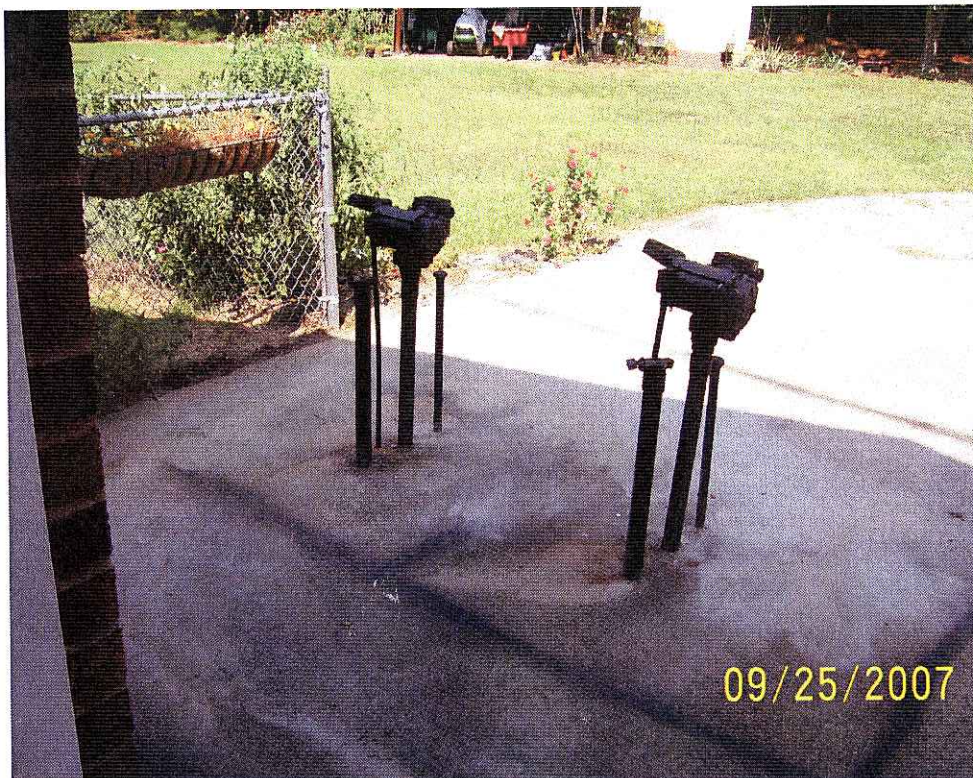
Photograph 2 – View of the two UST dispensers and fill ports.
