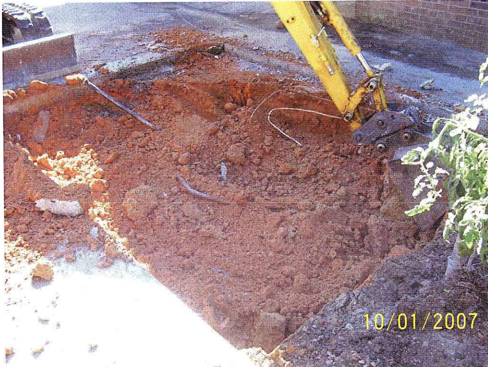
Photograph 3 - Preparing to remove the USTs.
