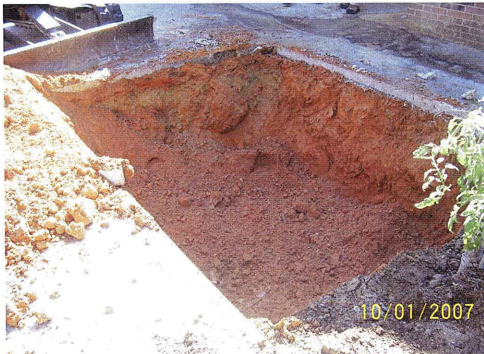
Photograph 8 – Excavation in the process of being backfilled.
