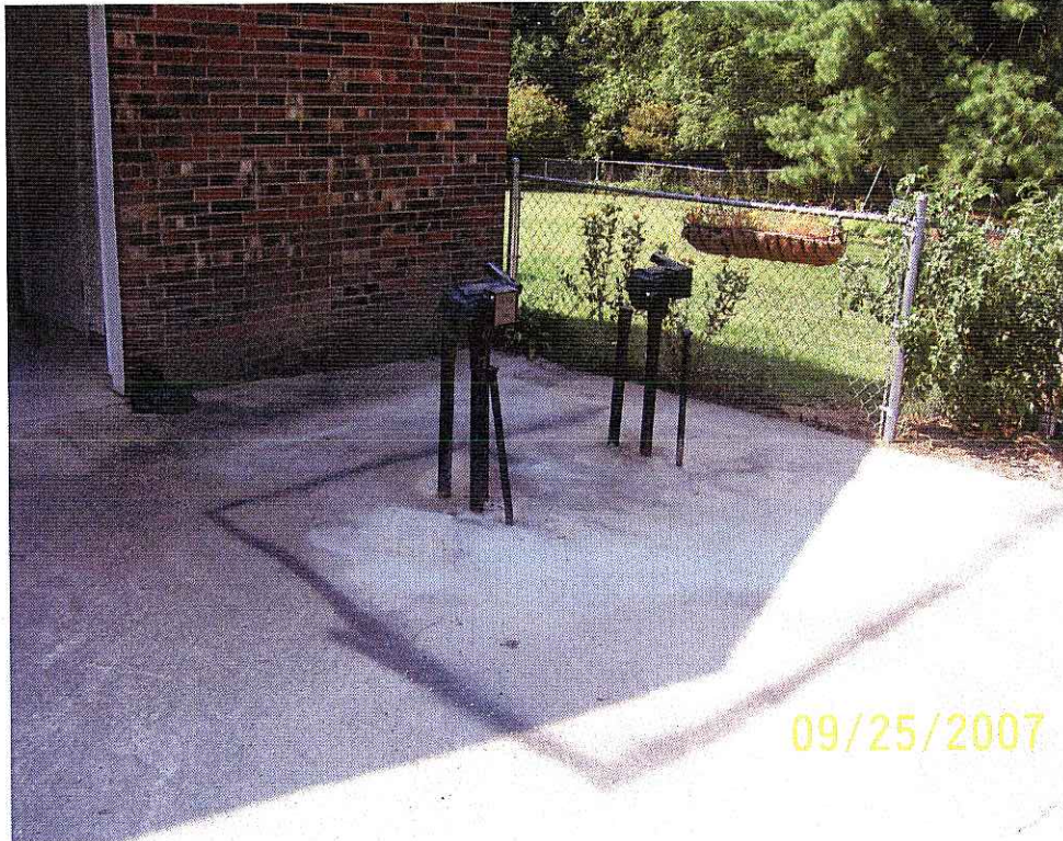
Photograph 1 – View of the two UST dispensers and fill ports.
