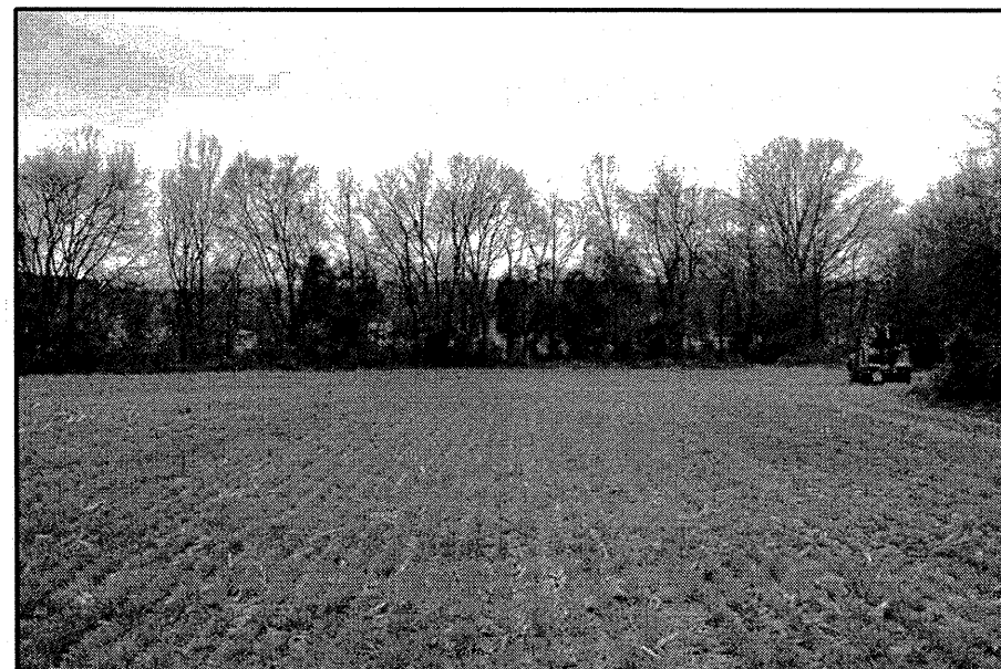
PHOTO TAKEN WITHIN EXISTING FIELD APPROXIMATELY 200 FEET NORTH (UPSTATION) FROM PROPOSED END BENT 2.
