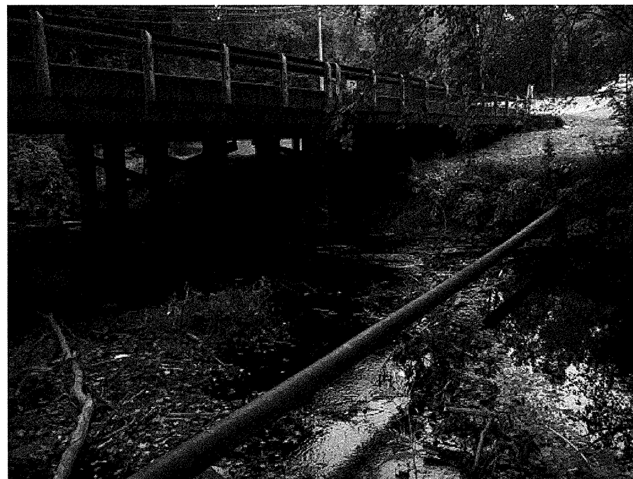
Photograph No. 2: View looking west at aerial sewer line and creek obstructions
