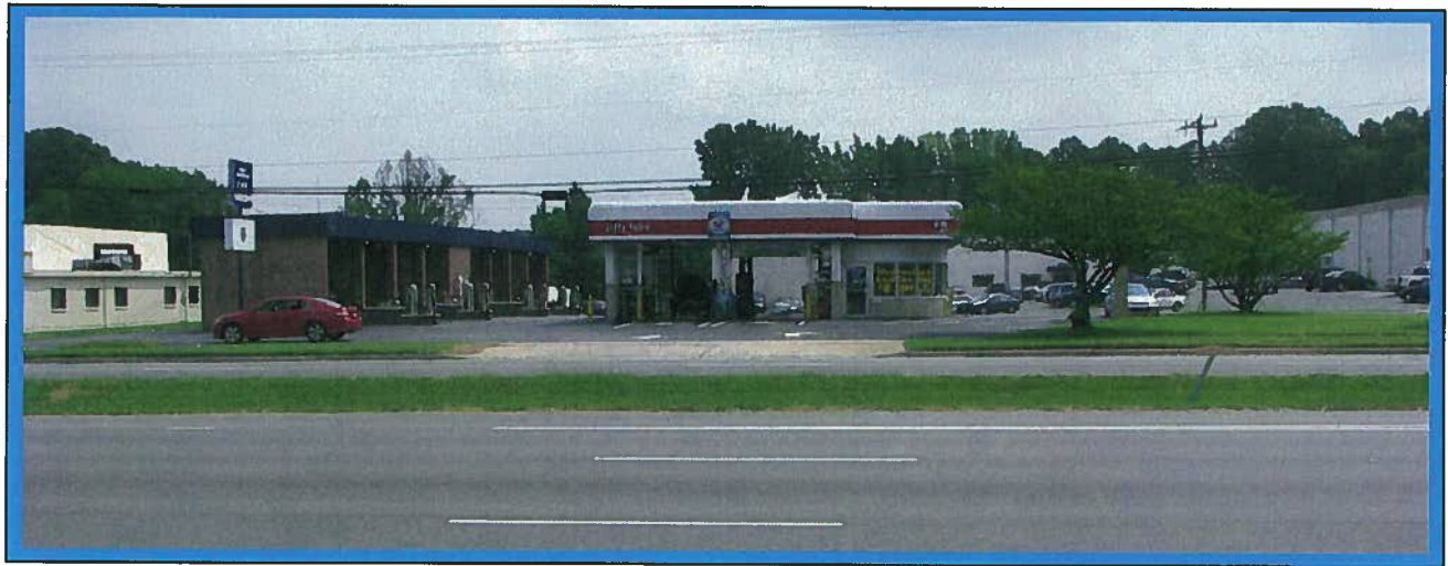
The photograph shows the southwestern (front) portion of the Hico Joan, LLC property located at the intersection of Independence Boulevard and Dion Avenue in Charlotte, North Carolina. The photograph is viewed in a northeasterly direction.
