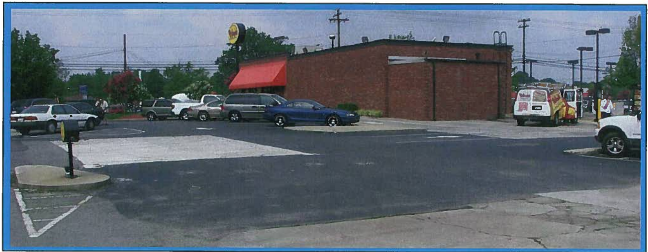
The photograph shows the back portion of the FFCA/IPI property located along the northerly side of Independence Boulevard in Charlotte, North Carolina. The photograph is viewed in a westerly direction.
