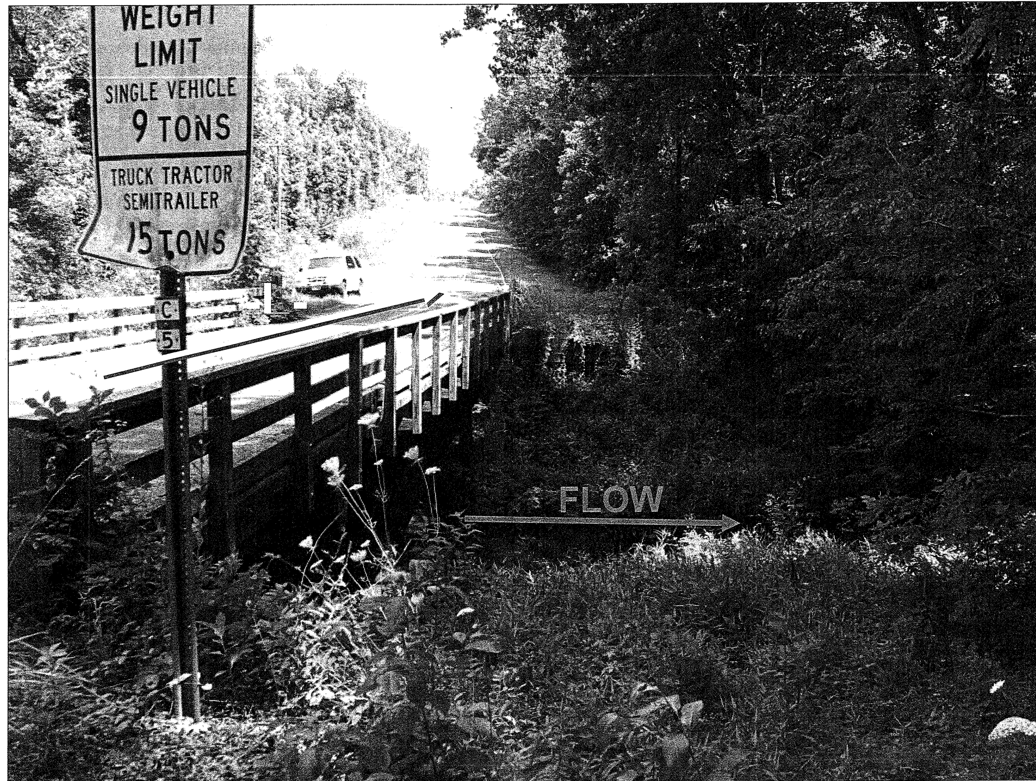
Looking North towards End Bent 2
