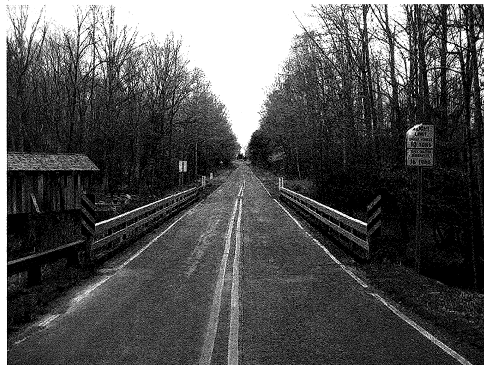
View looking west (down station)
