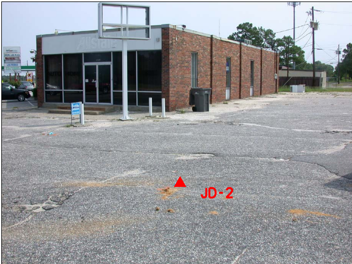
PHOTO 2 - BORING IN PROPOSED R/W LOOKING NORTHEAST
