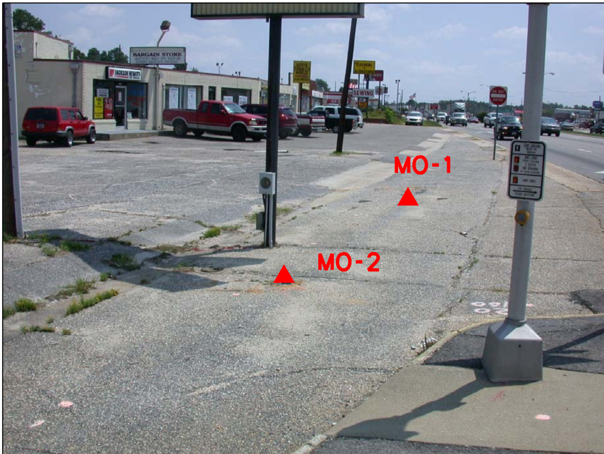
PHOTO 2 - BORINGS IN PROPOSED R/W LOOKING SOUTH
