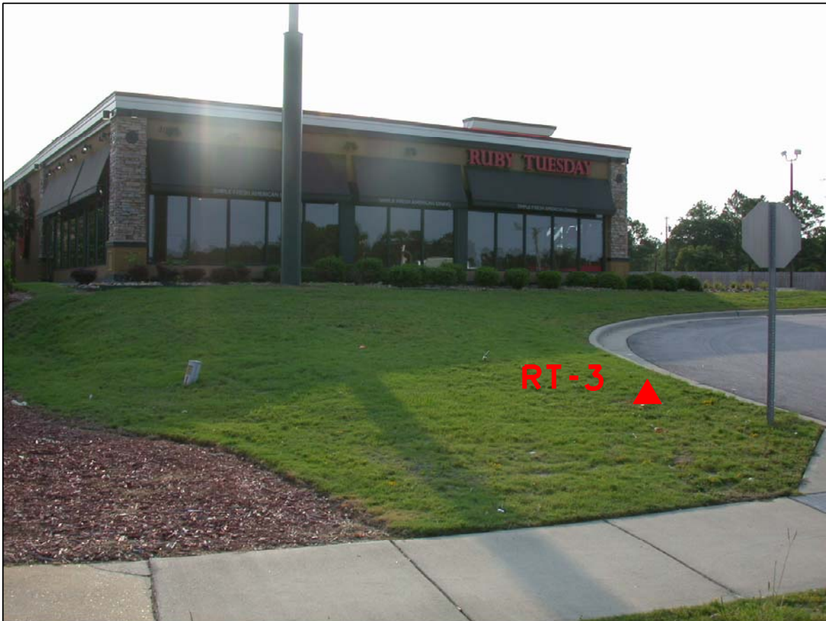
PHOTO 3 - BORING WITHIN PROPOSED R/W LOOKING EAST
