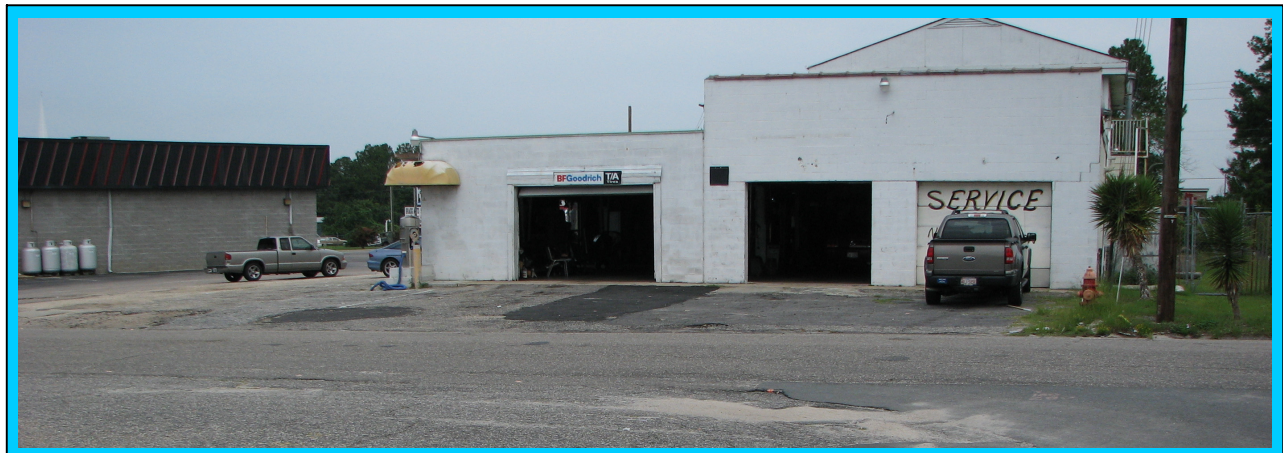
The photograph shows the proposed ROW area at the Willie Brantely site located along the northerly side of Wilson Avenue in Spring Lake, North Carolina. The photograph is viewed in a northwesterly direction.
