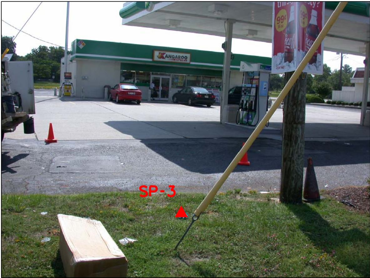
PHOTO 3 - BORING WITHIN PROPOSED R/W LOOKING EAST
