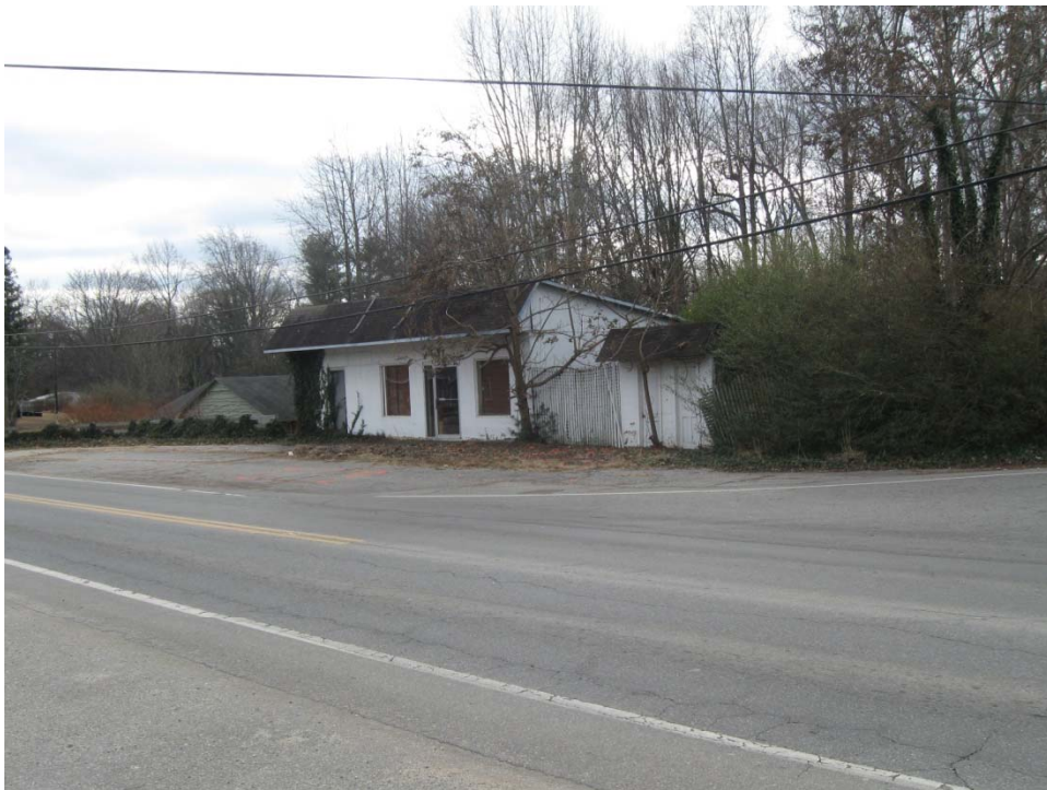
Parcel 87 – Olaf and Valeria Adams Property, looking southwest
