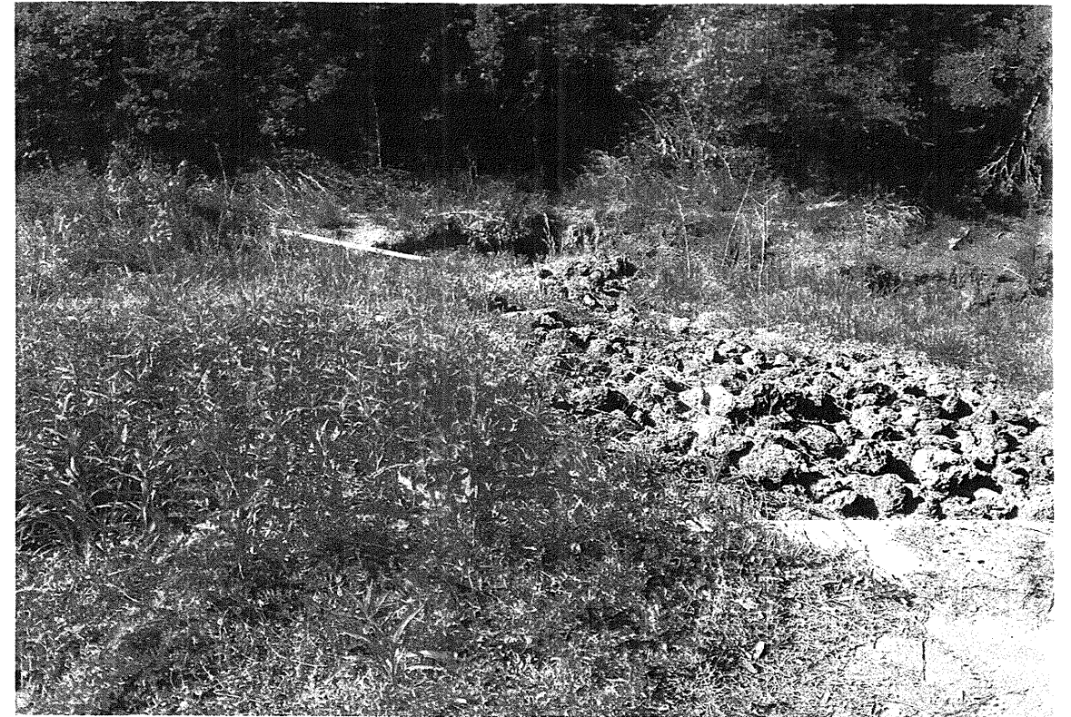
View looking left to right of End Bent No. 2
