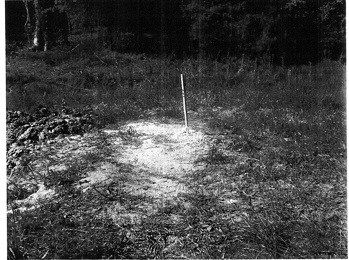
View looking left to right of End Bent No. 1
