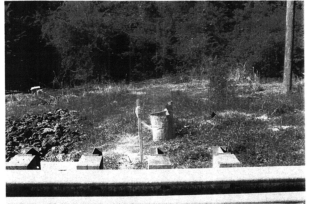
View looking left to right of Interior Bent No. 4
