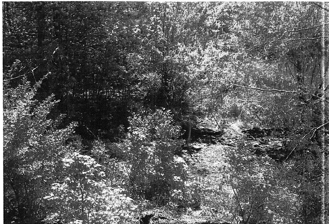
View looking right to left of End Bent No. 1
