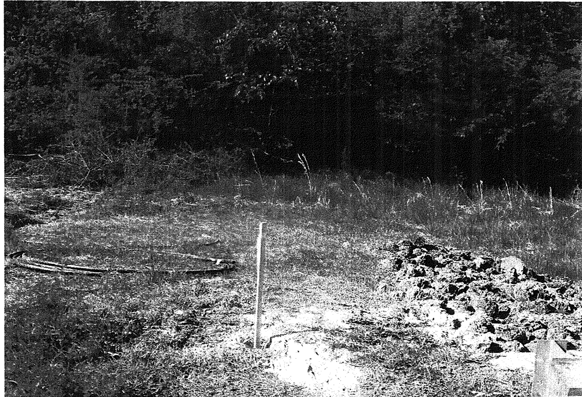
View looking left to right of Interior Bent No. 2
