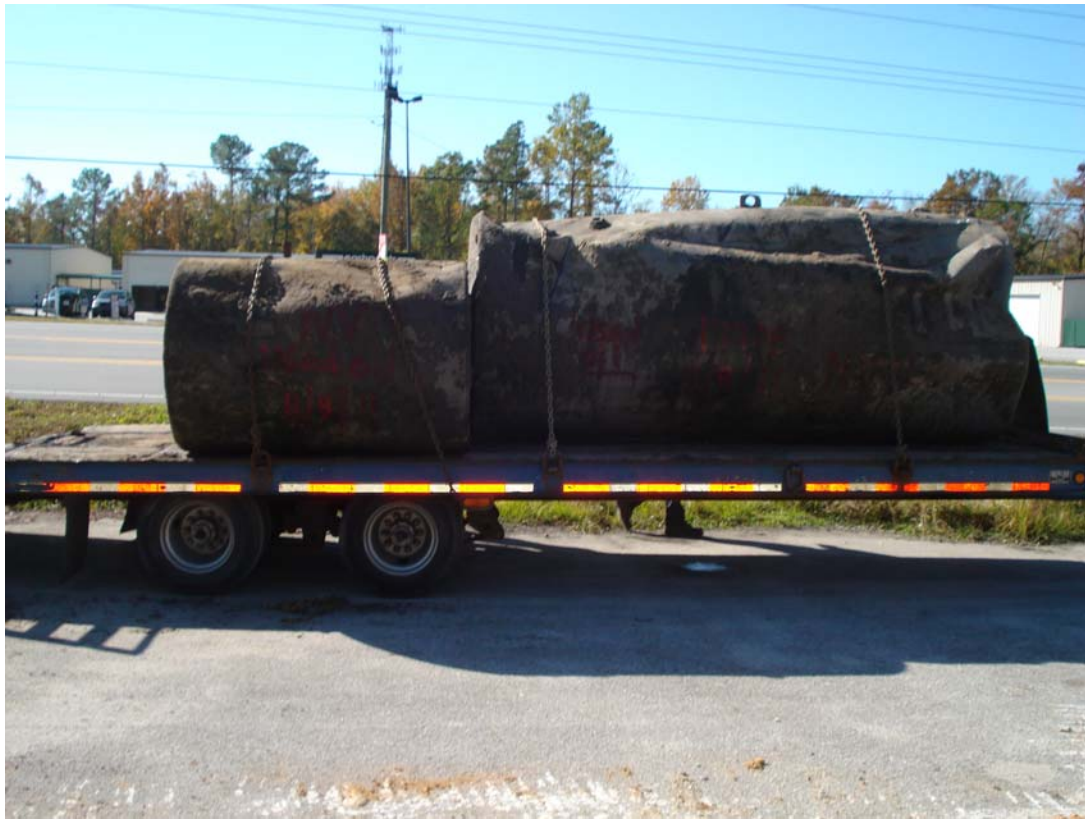
Photograph 6: UST #001 (on right) and UST #002 (on left) loaded for offsite disposal.
