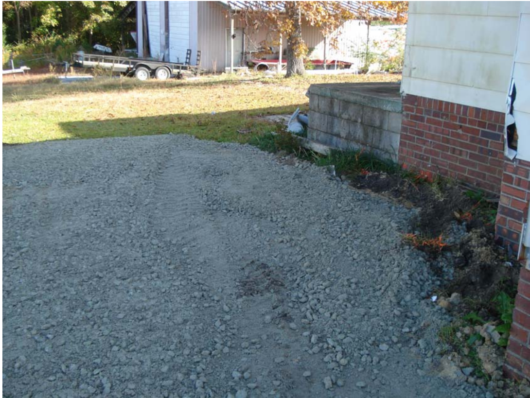
Photograph 10: View looking northeast at backfilled and compacted UST #003 excavation.
