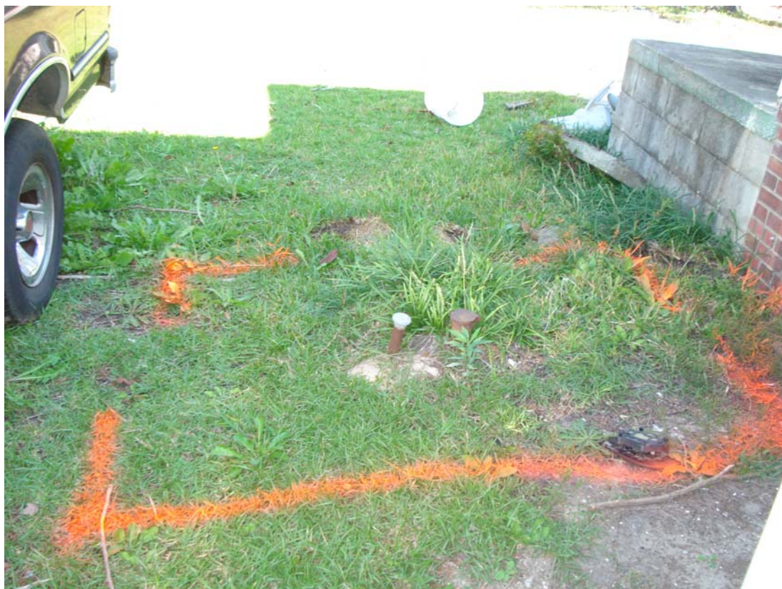
Photograph 2: View looking north at UST #003 prior to removal.
