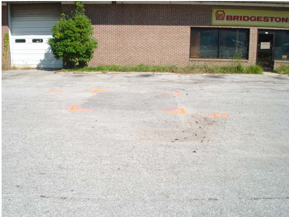
Photograph 1: View looking north at location of USTs #001 and #002 prior to removal.
