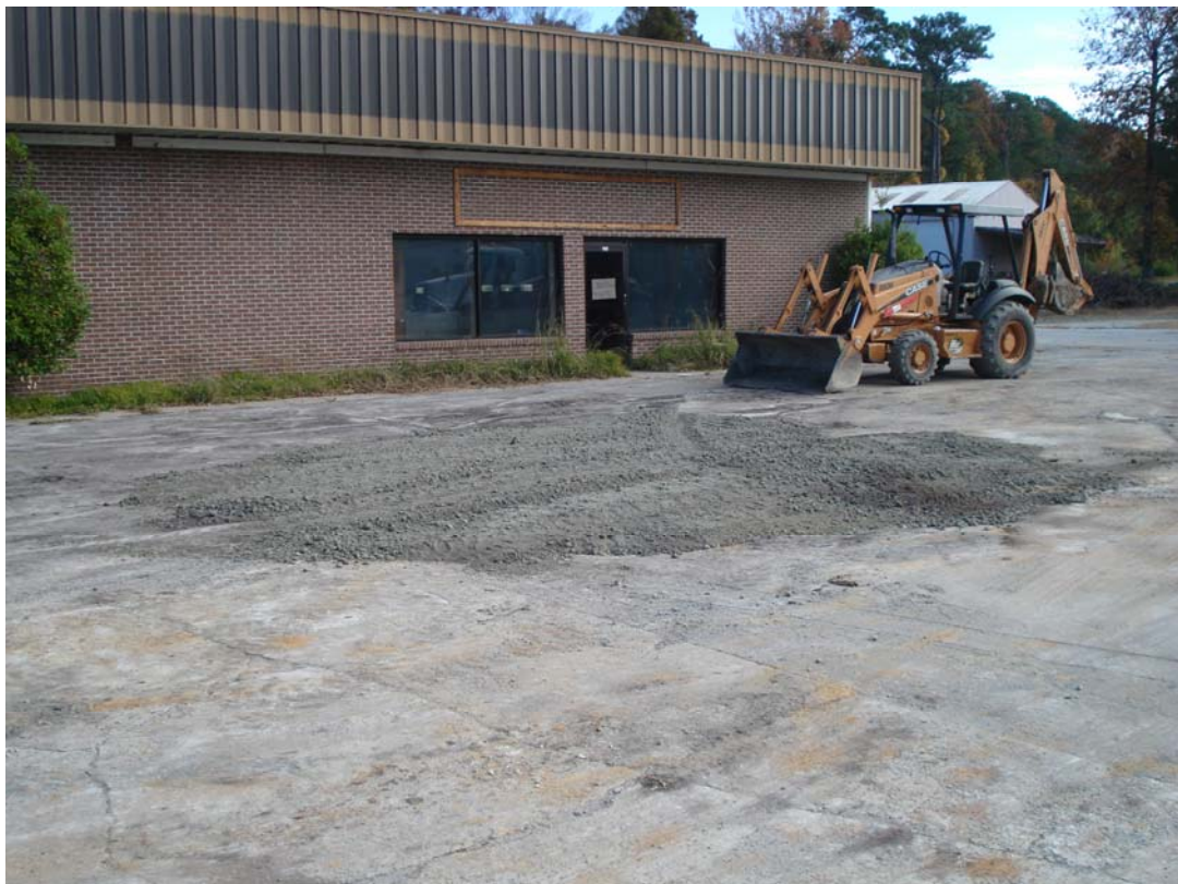
Photograph 9: View looking northeast at backfilled and compacted UST #001/#002 excavation.
