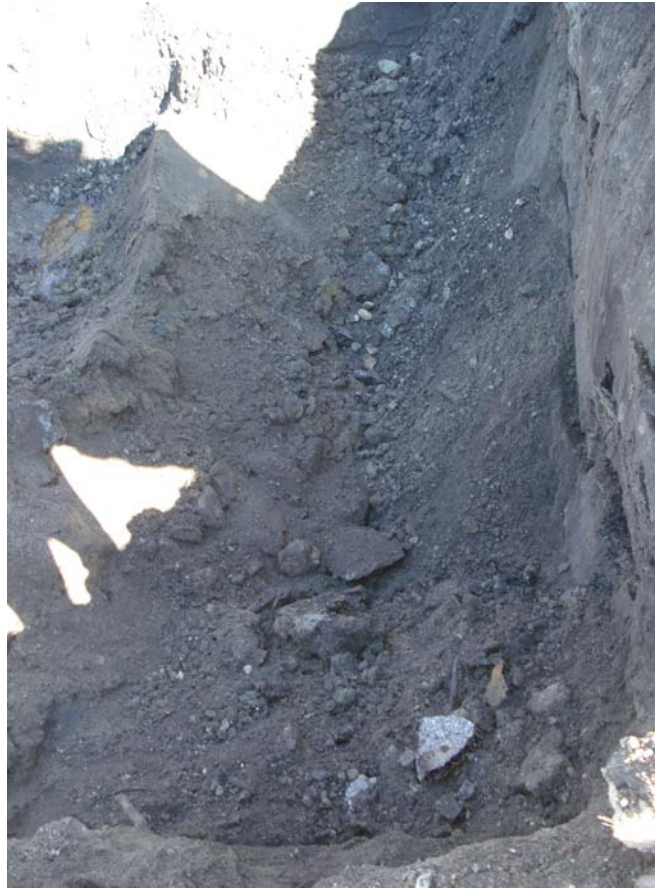
Photograph 3: View looking north at former location of UST #001 prior to overexcavation.
