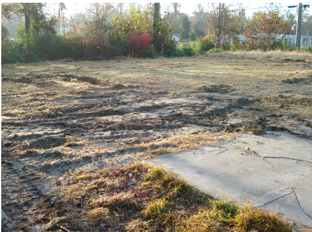
Photograph 3: View looking south at UST excavation following backfilling and compaction.
