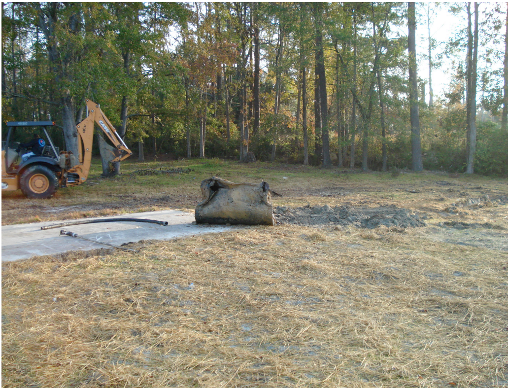
Photograph 2: View looking east at heating oil UST following removal.
