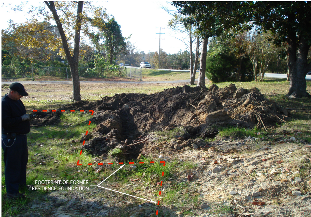
Photograph 3: View looking south at completion of excavation activities.
