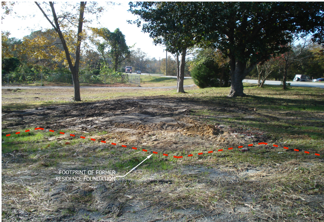
Photograph 4: View looking southwest at excavation area following regrading.
