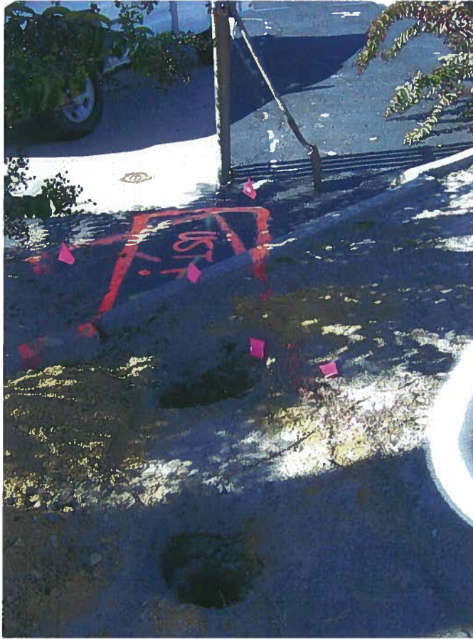
Photograph 5– View looking west corresponding to the possible UST noted in the geophysical report.
