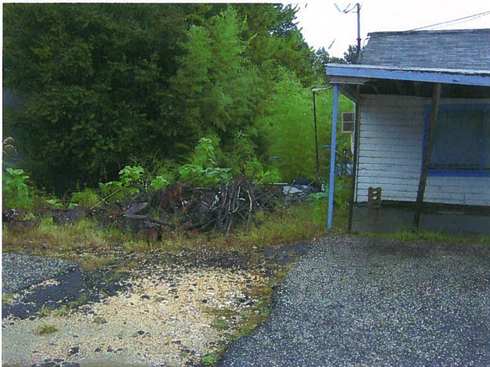
Photograph 2 – View looking east along the north side of the building.
