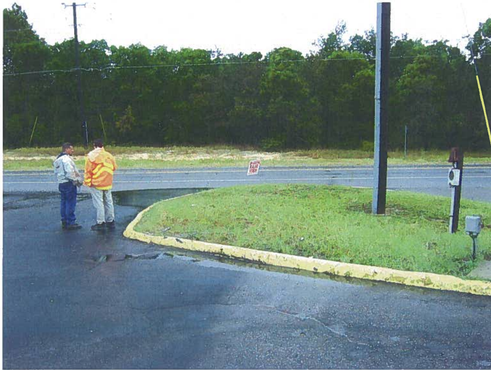
Photograph 1 – View looking east at area of future DOT drainage
