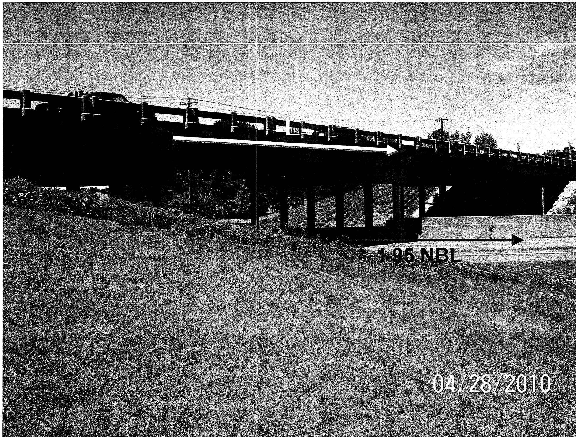
Looking Southwest towards End Bent 2
