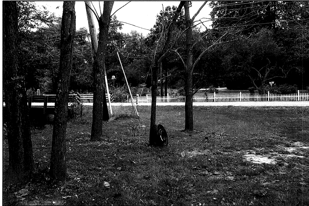
PHOTO 3: END BENT 1, LOOKING FROM LEFT TO RIGHT.
