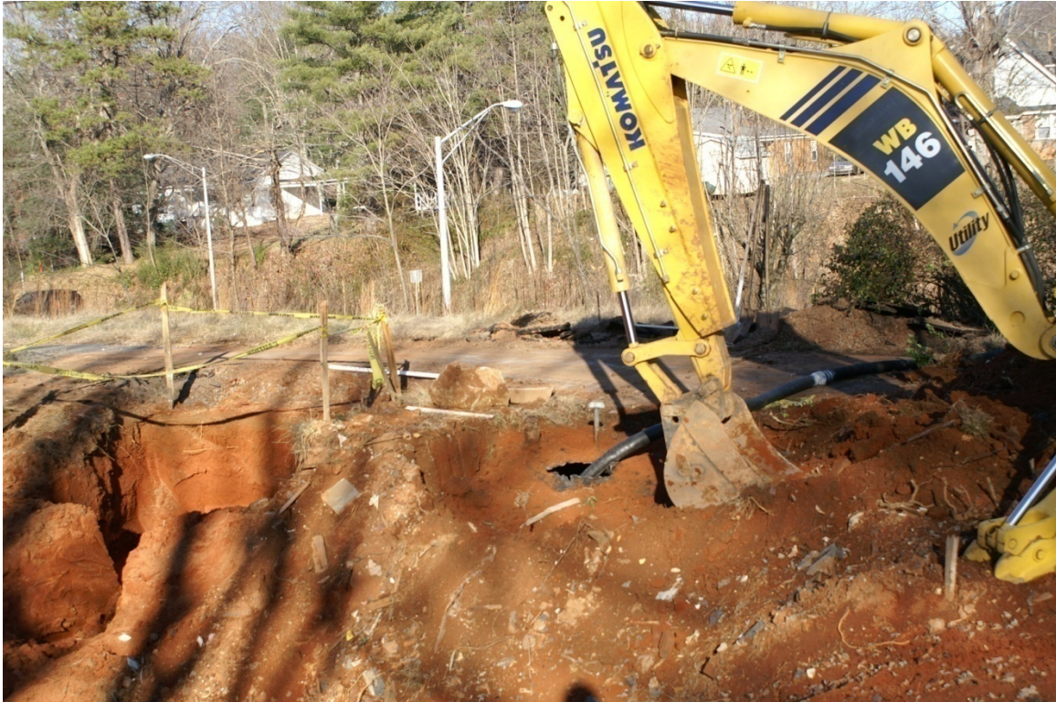
Photograph 1: Removal of residual material from UST (view to the northeast).
