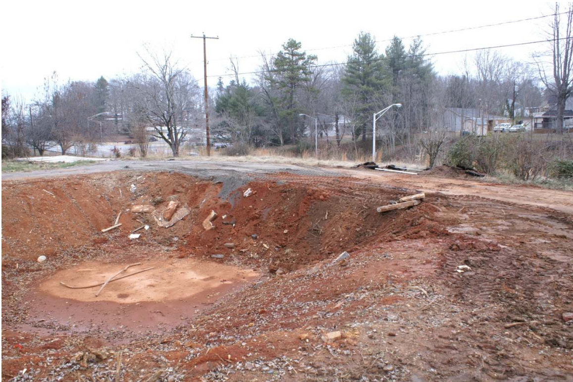
Photograph 6: Area of UST removal after completion of backfilling activities (view to the northeast).
