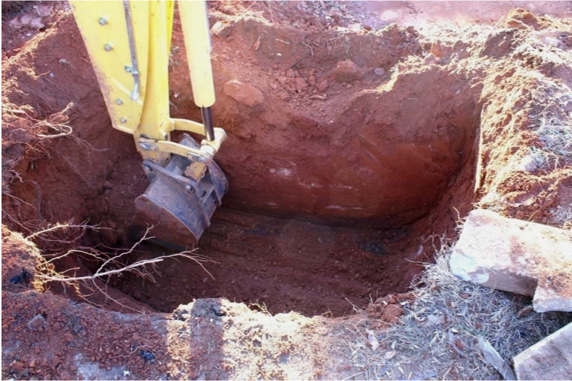
Photograph 5: View of over-excavation activities (view to the west).
