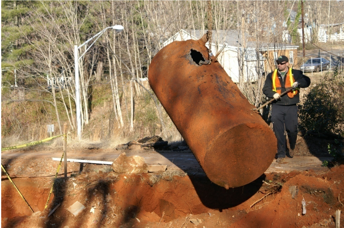
Photograph 2: Removal of UST (view to the east).
