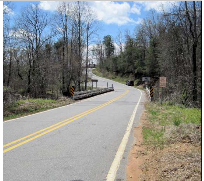
Bridge 38 over Jacob Fork River on SR 1901 (Wards Gap Road). View to the southwest.
