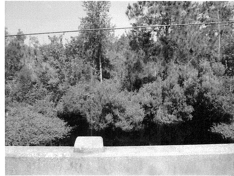
Photograph No. 11: This photograph was taken from the right side of the -L- alignment, looking west, across proposed Interior Bent No. 6.
