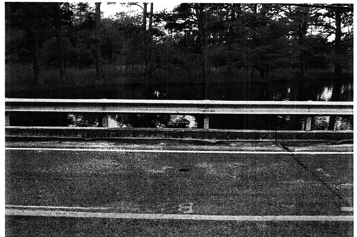
Interior Bent No. 1: View Looking Right to Left.
