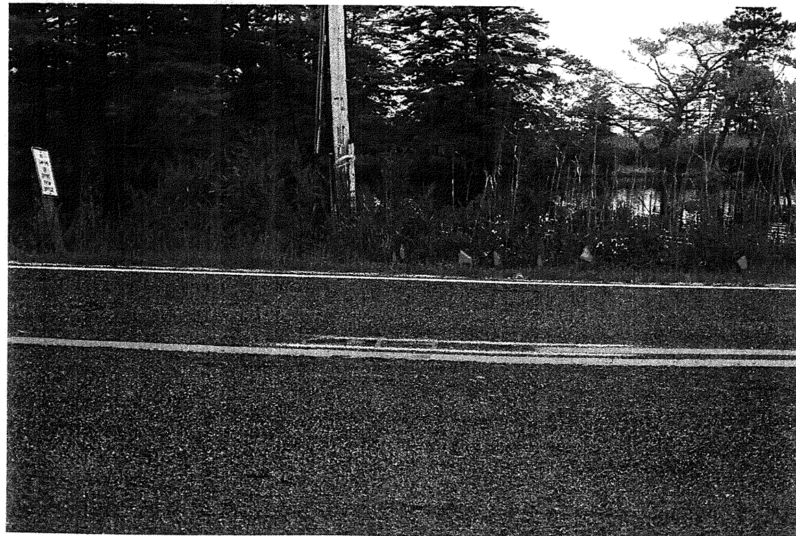
End Bent No. 2: View Looking Right to Left.
