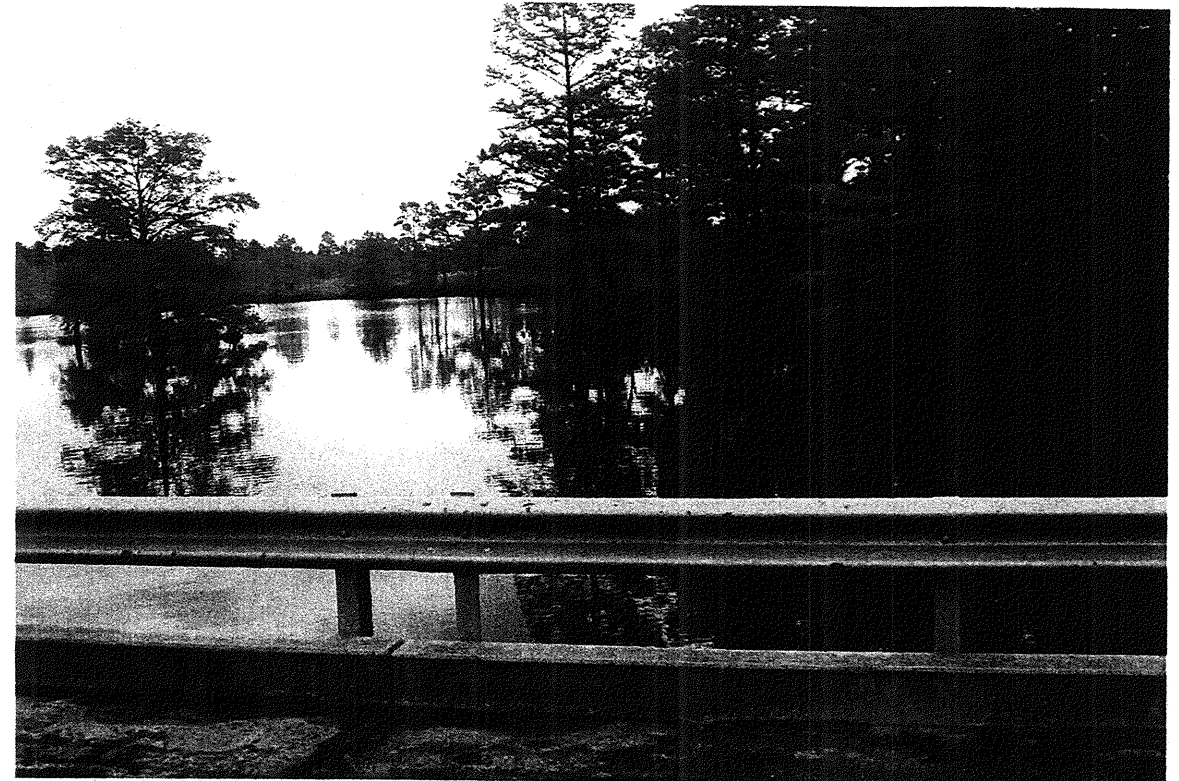
View From Existing Bridge Looking Upstream
