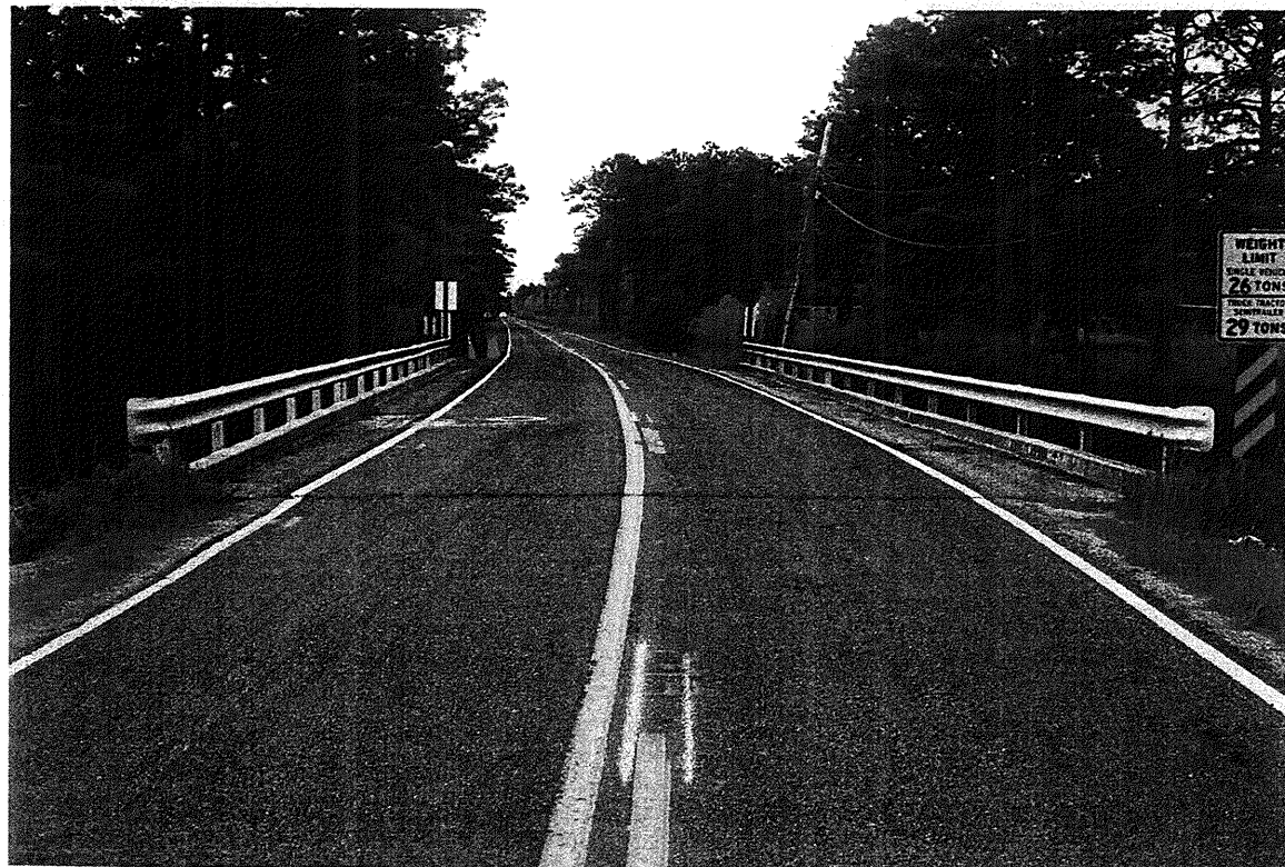
View Looking Down Station from End Bent No. 2
