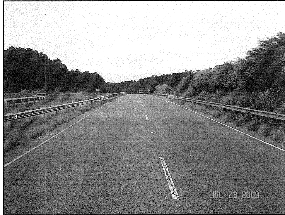
PHOTOGRAPH No. 1: Taken from the northeast approach of the replacement bridge End Bent #1, along the -L- alignment, looking southwest, at the existing bridge
