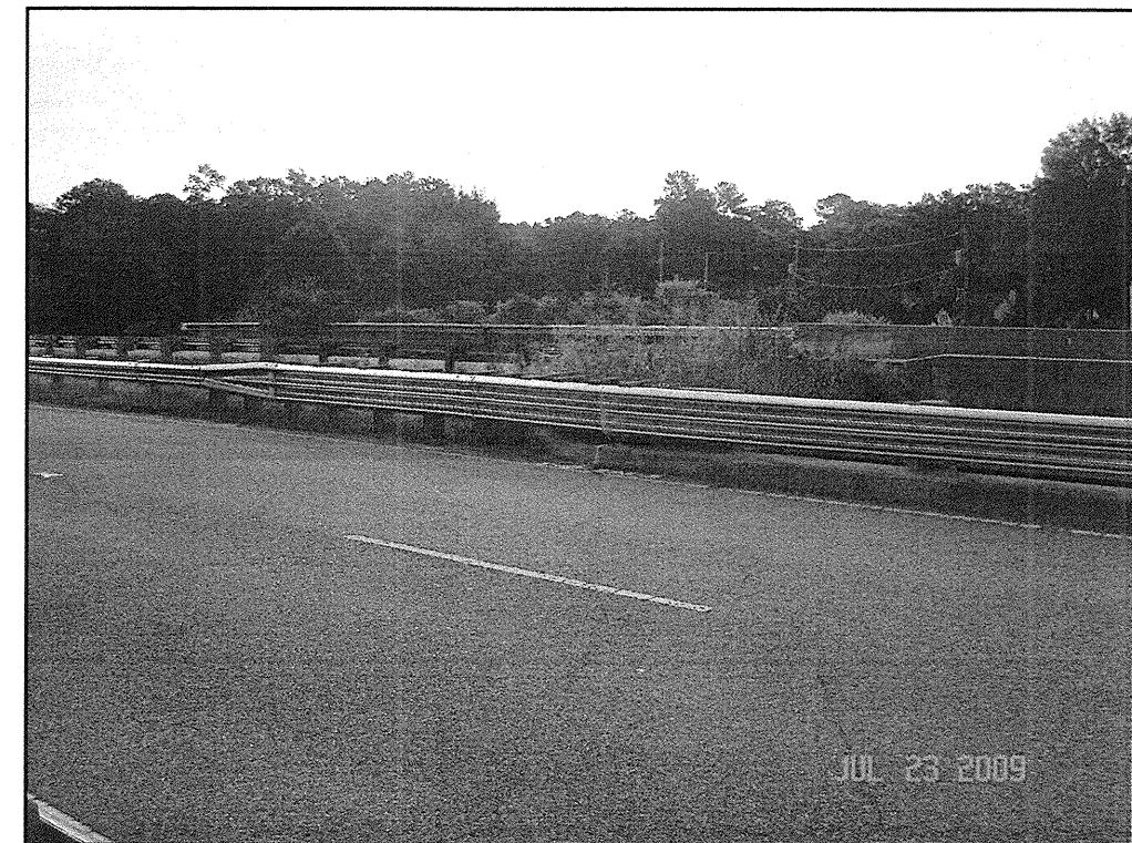
PHOTOGRAPH No. 4: Taken from the left side of the -L- alignment, looking east across proposed End Bent #2 of the replacement bridge
