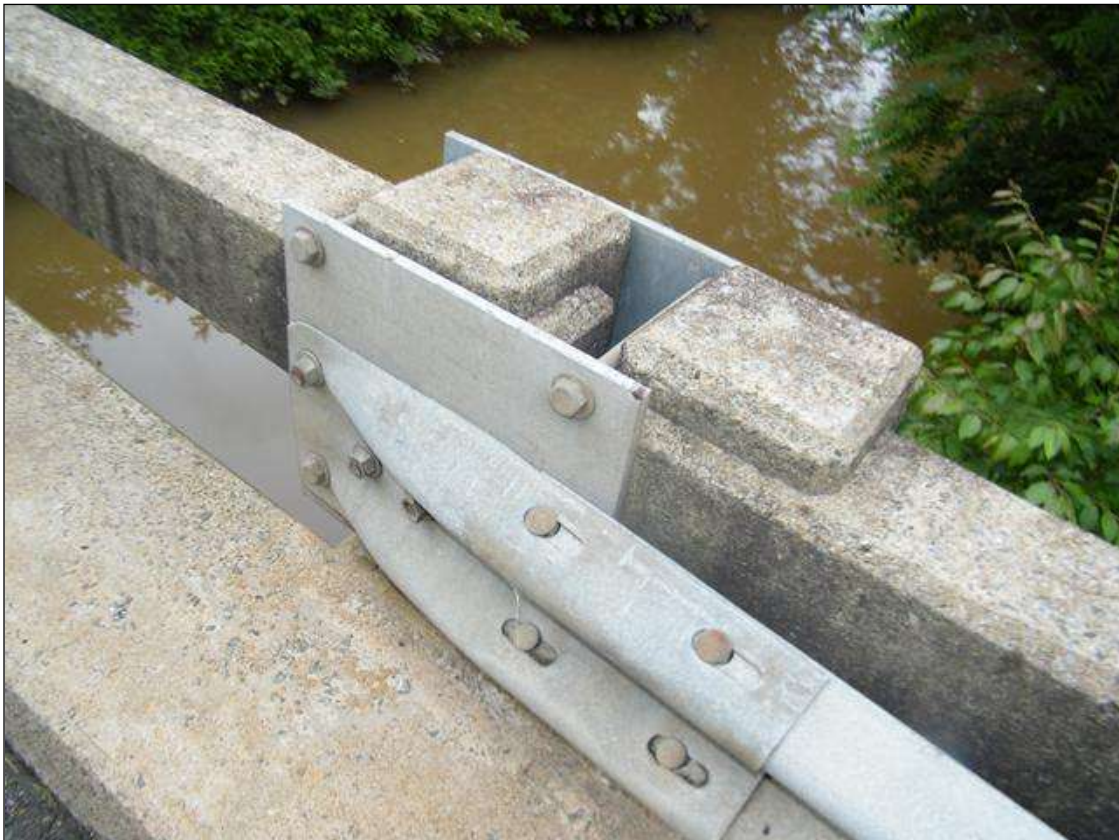
GUARDRAIL ATTACHMENT
