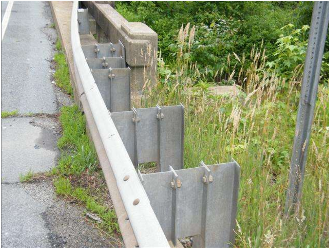
GUARDRAIL SPACING AT BRIDGE
