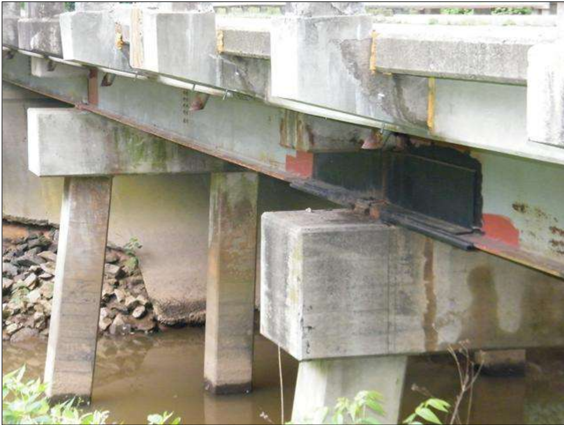
BEAM AT END OF CAP
