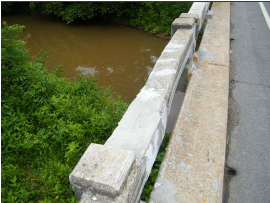
RIGHT RAIL HAS BEEN REPAIRED
