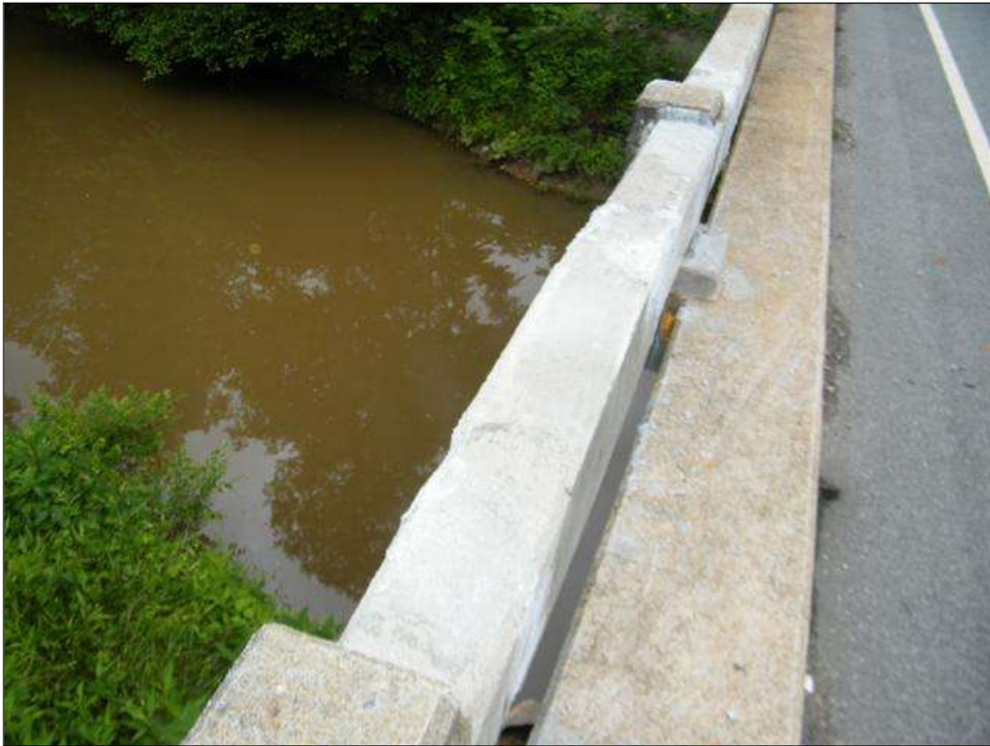
RIGHT RAIL HAS BEEN REPAIRED
