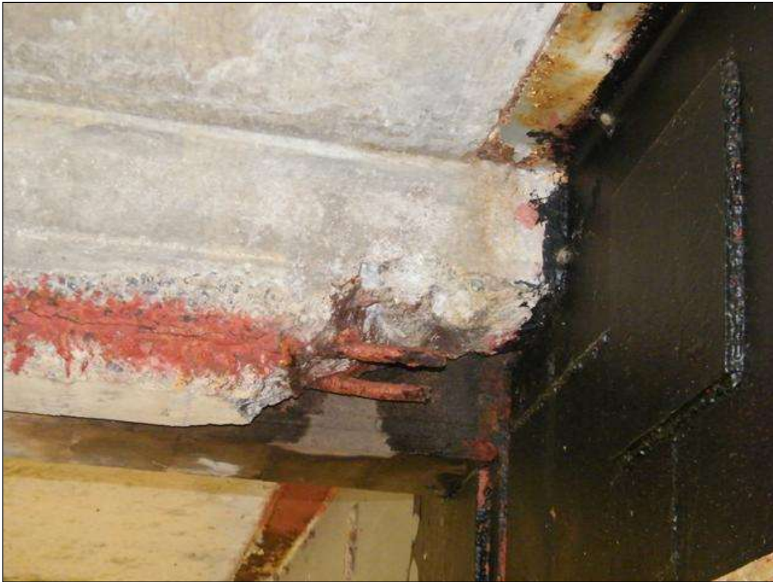
END DIAPHRAGMS HAVE BEEN CUT TO REPAIR BEAMS AT PIER 2
