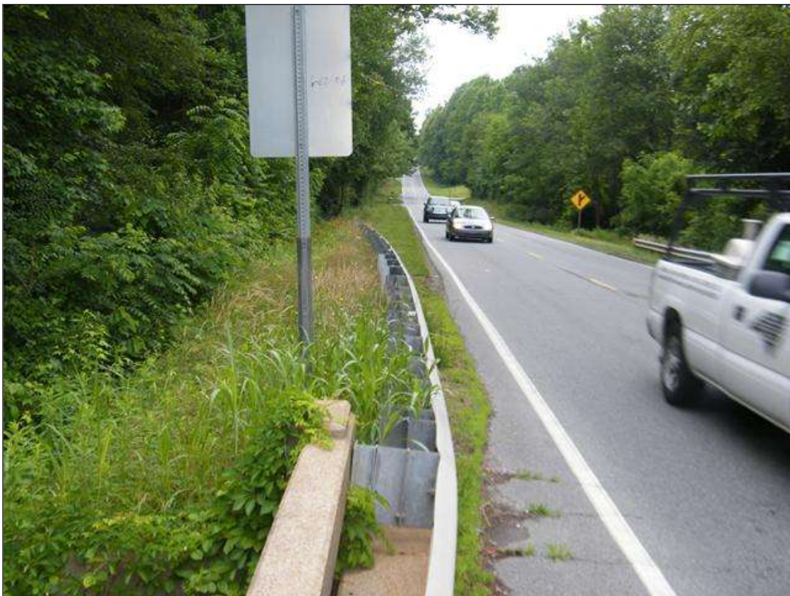
GUARDRAIL LOOKING NORTH
