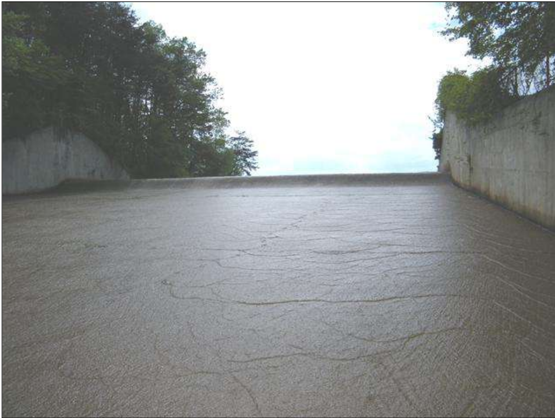
LOOKING WEST UPSTREAM
