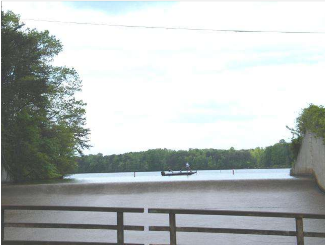
LOOKING WEST UPSTREAM FROM TOP
