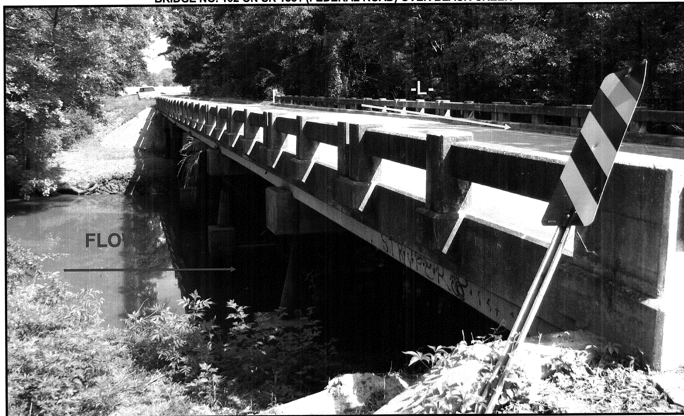
LOOKING NORTH TOWARD END BENT 1
