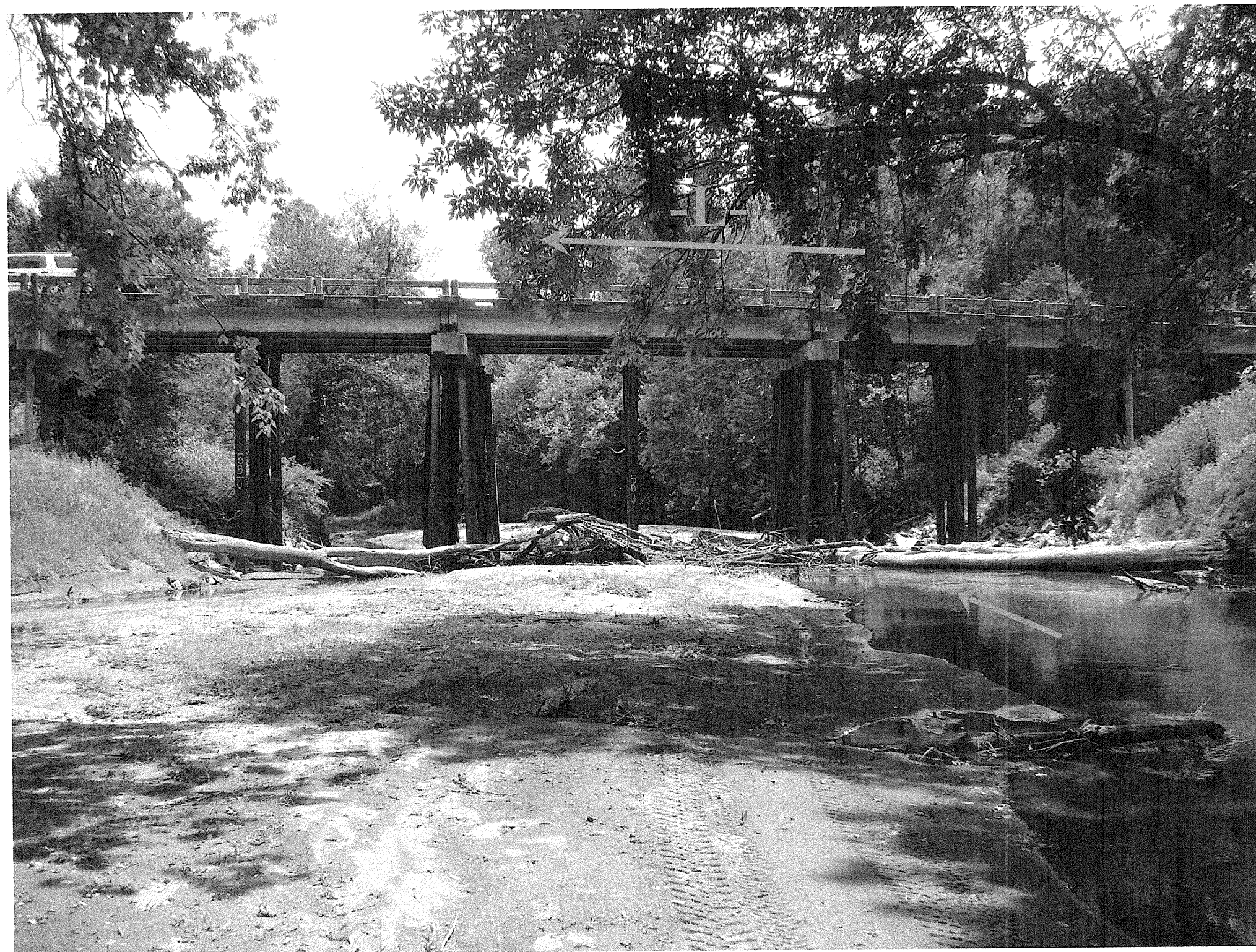
Looking Southeast downstream
