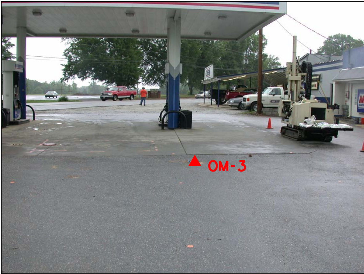
PHOTO 3 - BORING WITHIN PROPOSED R/W LOOKING NORTH
