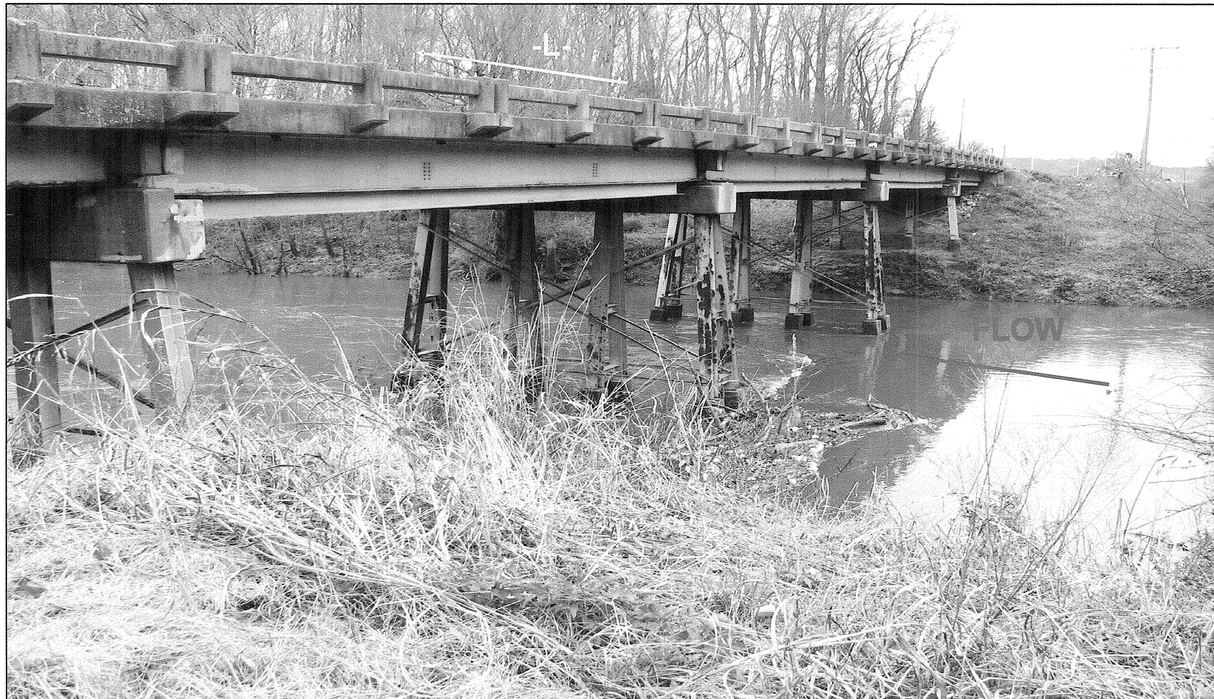
LOOKING EAST TOWARD END BENT 1
