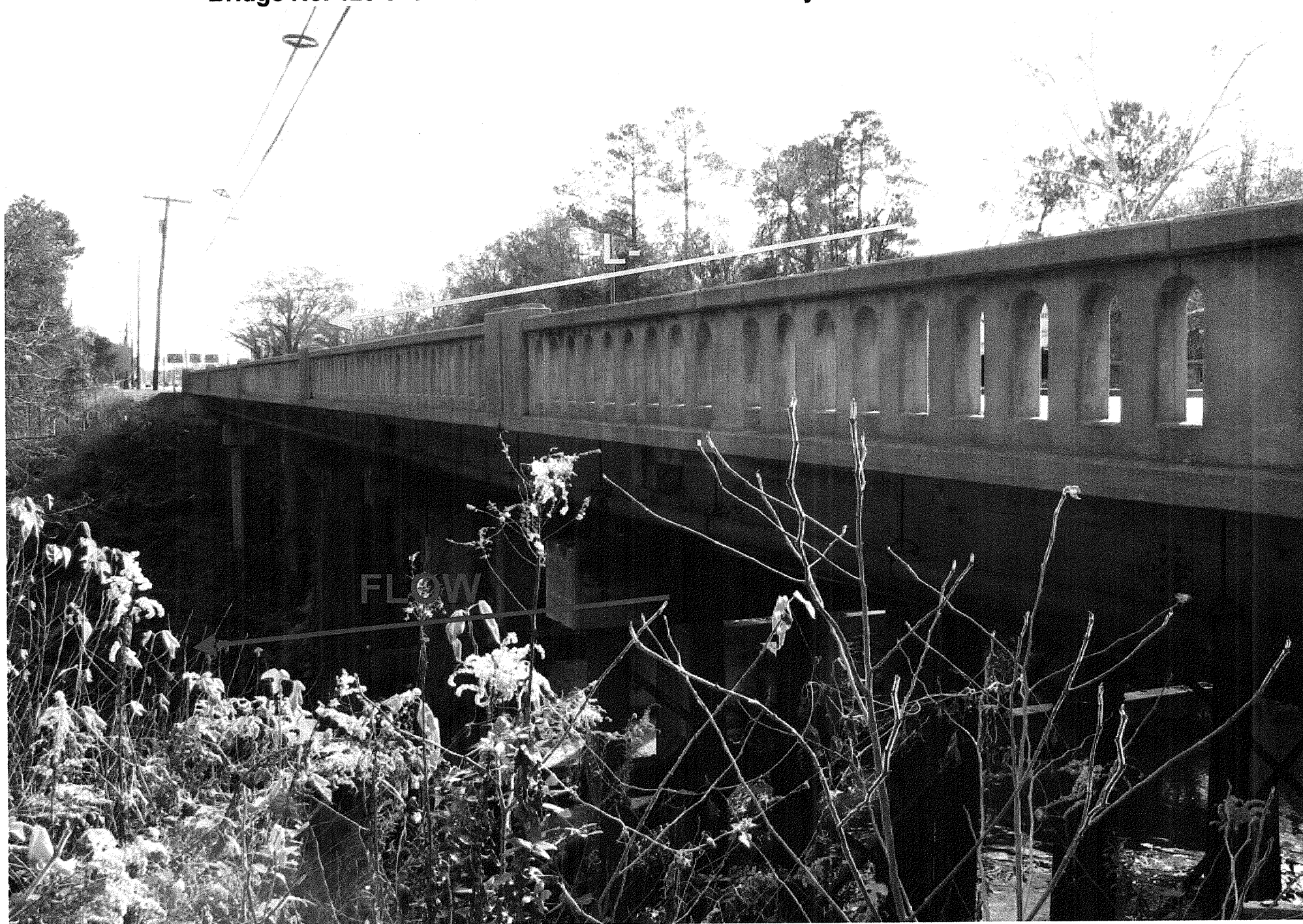
Looking East toward End Bent 2
