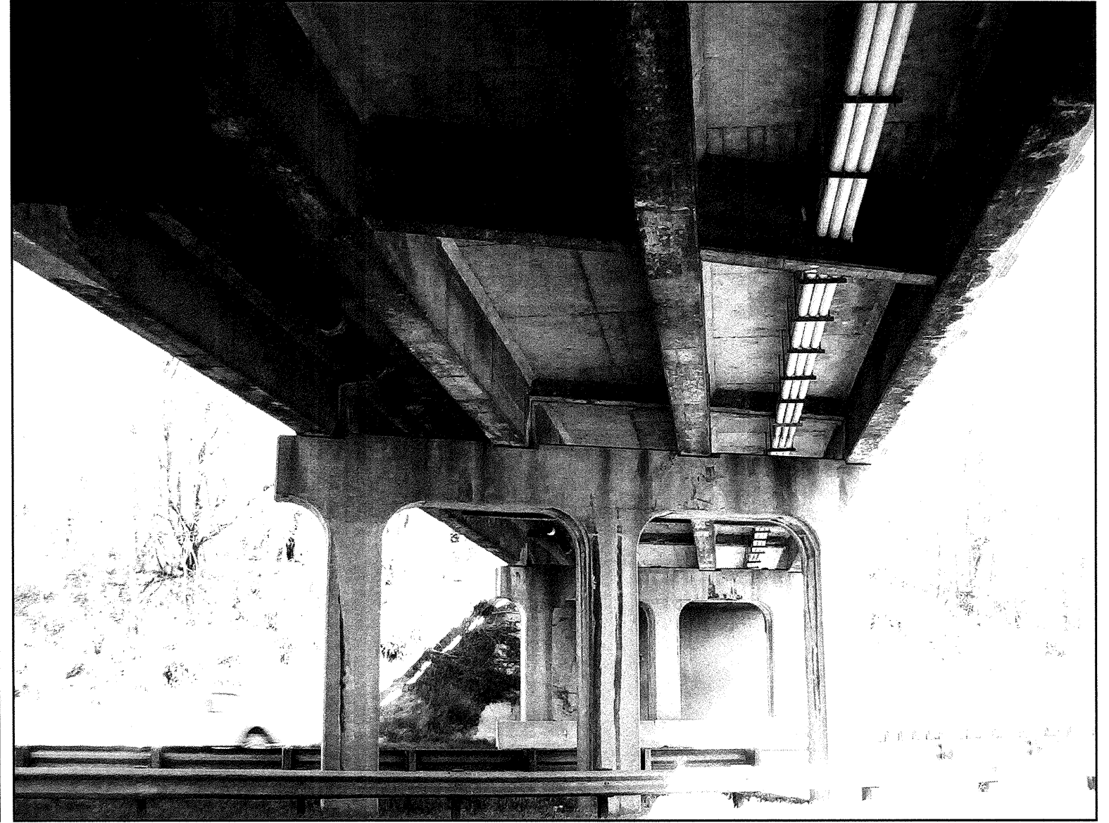
LOOKING NORTH (UPSTATION) TOWARDS BENT 1 FROM TOE OF EXISTING END BENT 1 SLOPE.
