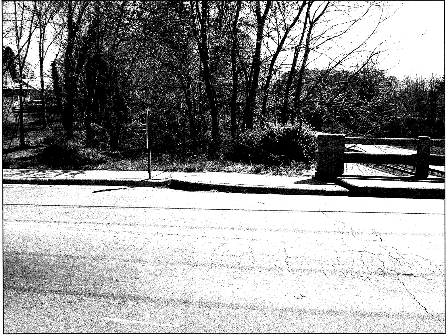
LOOKING EAST (RT) ALONG END BENT 2.
