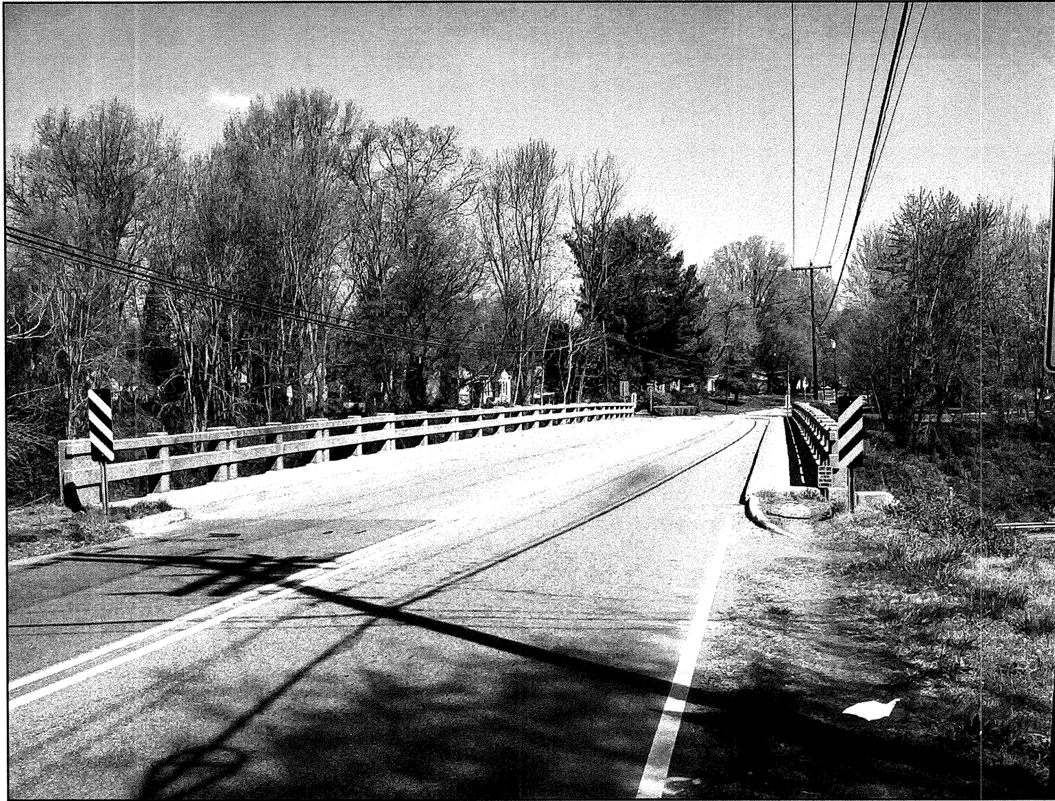
OVERVIEW OF EXISTING BRIDGE, LOOKING NORTH (UPSTATION) FROM END BENT 1.
