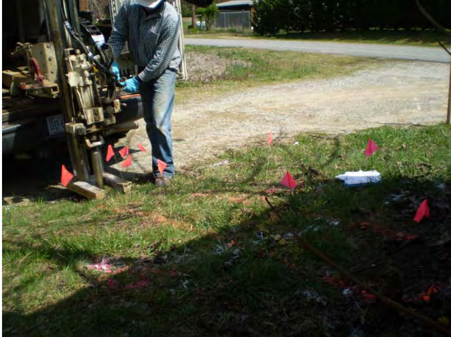
Photograph 3 – View of geophysical mark out of probable segment of wide-diameter conduit, culvert or possibly a small metallic UST behind the north-east corner of the art gallery.
