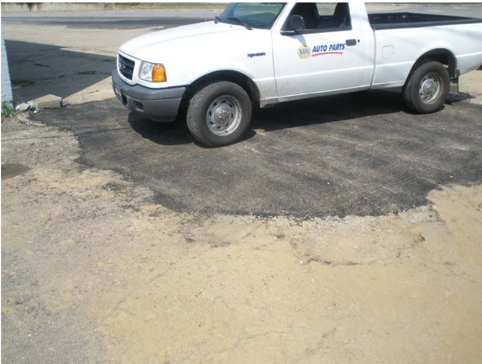
Photograph 6: View northwest at newly-applied asphalt paving over UST excavation.
