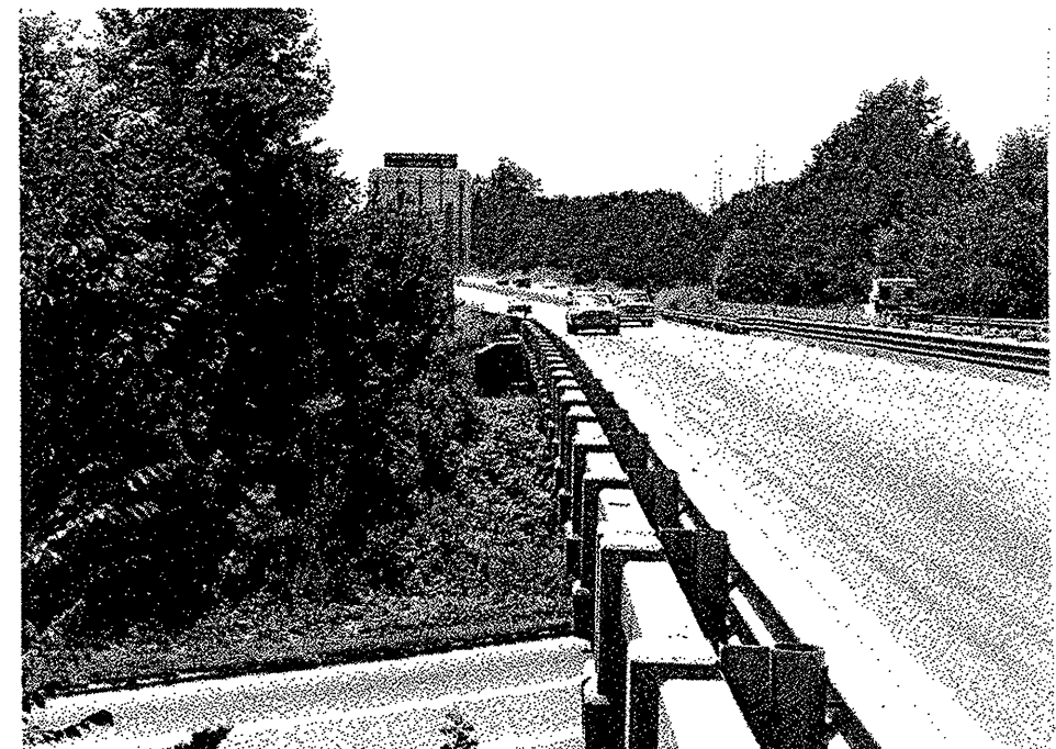
LOOKING WEST ALONG RIGHT STRUCTURE PARALLEL TO -Y26- LINE (I-40)
