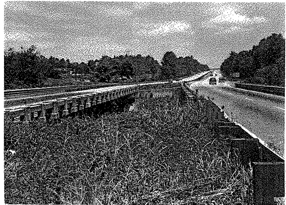
LOOKING EAST FROM END BENT-1 ALONG -Y26- LINE (I-40)
