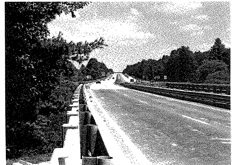
LOOKING EAST ALONG LEFT STRUCTURE PARALLEL TO -Y26- LINE (I-40)
