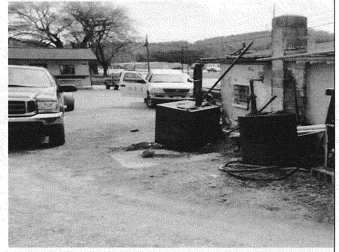
Photograph 4: Rear of the site building. Note waste oil UST location, kerosene dispenser, and apparent leaking oil cube.
