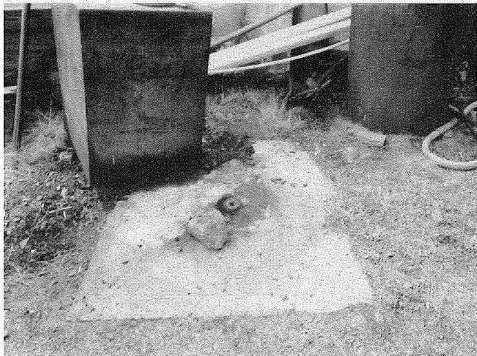
Photograph 5: Close up view of UST and apparent leaking oil cube situated beyond the NCDOT Right-of-Way. Note
