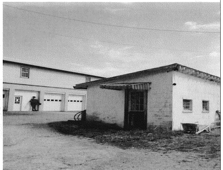
Photograph 2: A closer view from the northwest.
