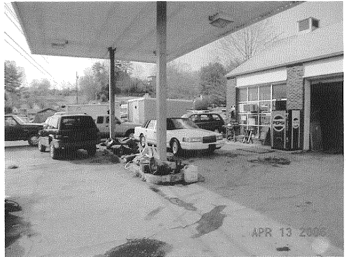
Photograph 2: View of former pump island fronting site building, beyond which is the location of former USTs.
