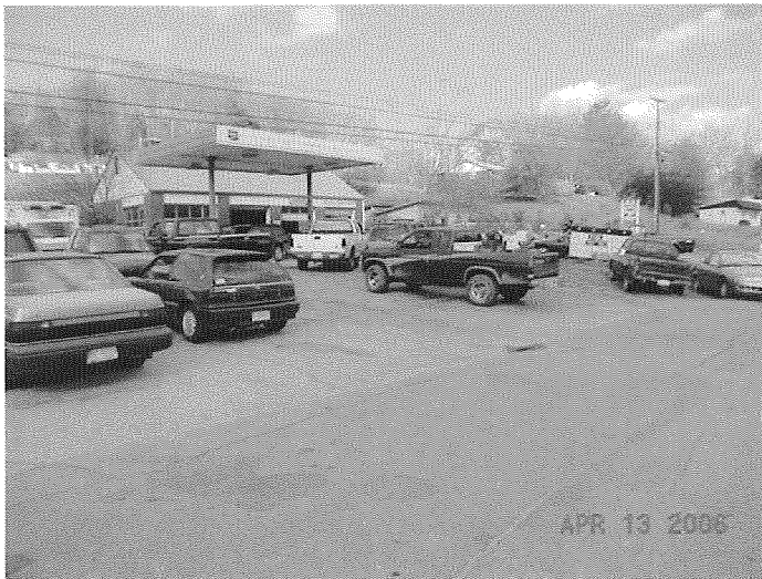
Photograph 1: View of subject property area of investigation adjacent to Austin Automotive.
