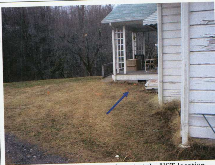
Photograph 4: Looking southwest at the UST location.
