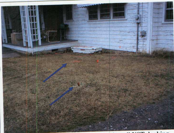
Photograph 3: Another view of heating oil UST, looking northwest. Flags in this photo mark a local u/g water line.
