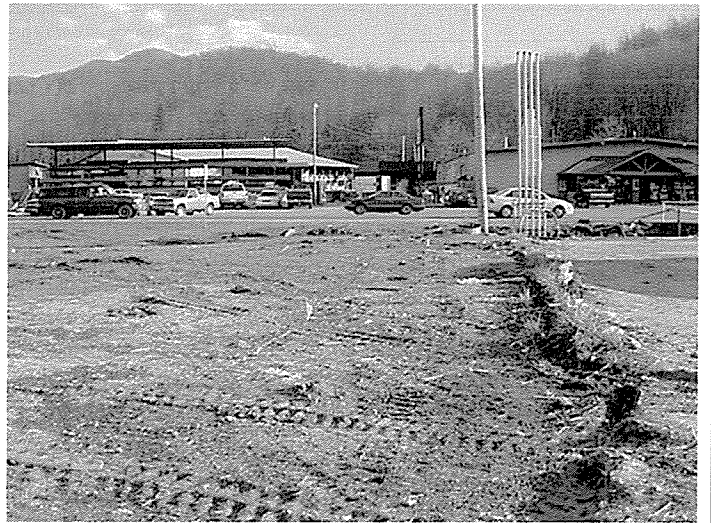
Borings GP1-GP3 and GP7 facing south
