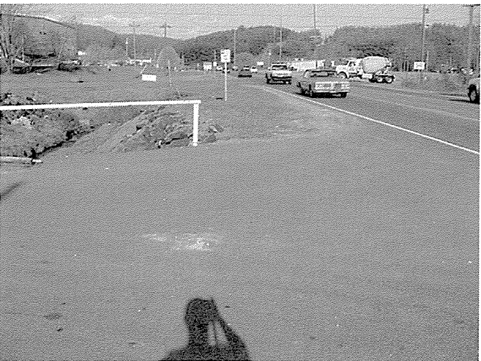
Boring GP9-GP11 facing east
